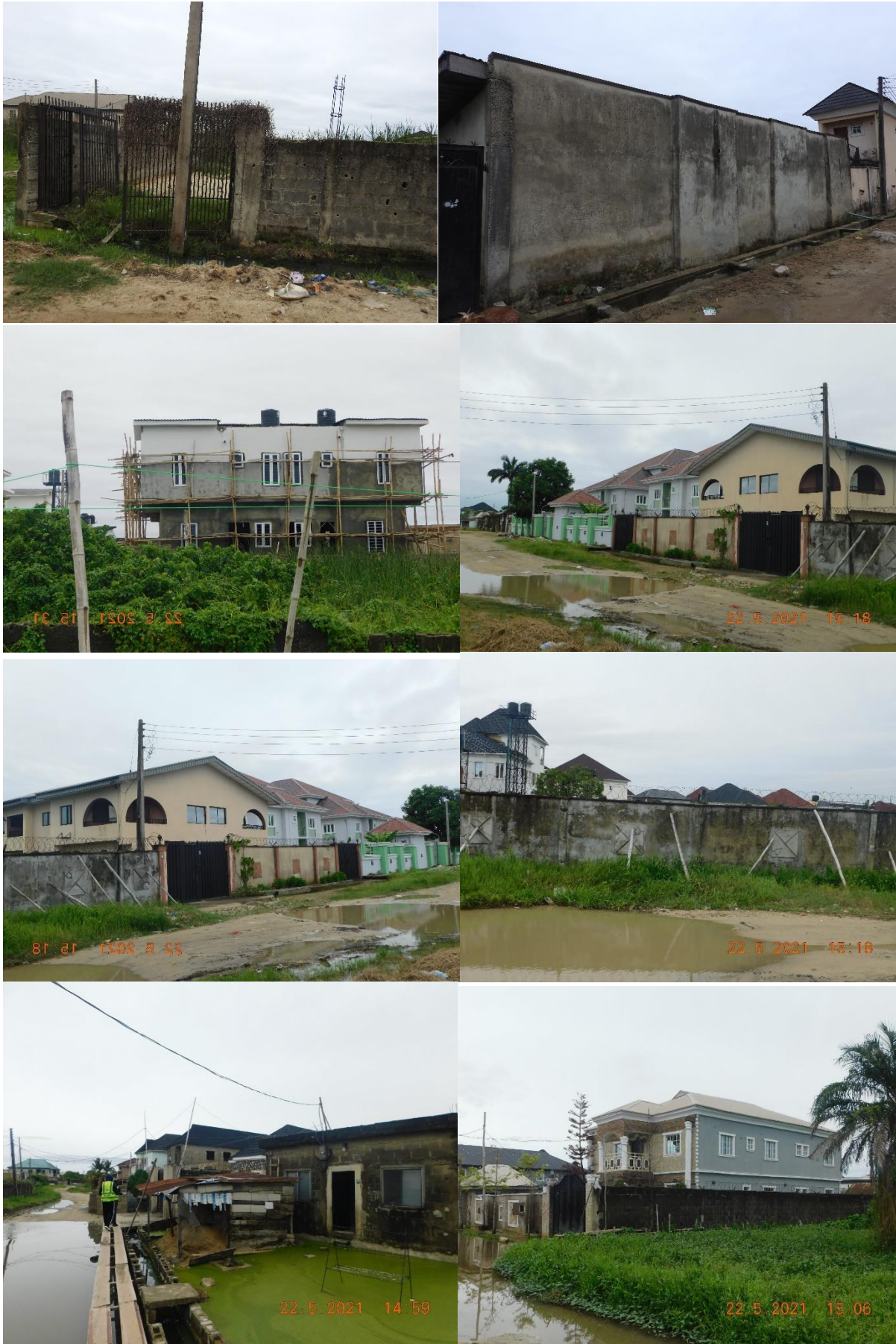
Plate 7.3: Pictures of potential affected structures at Power line area, Ajah, Lagos
