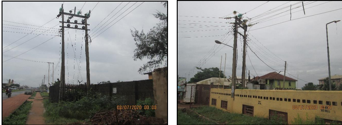
Plate 4.16: Electricity Infrastructure Observed in the Study area
