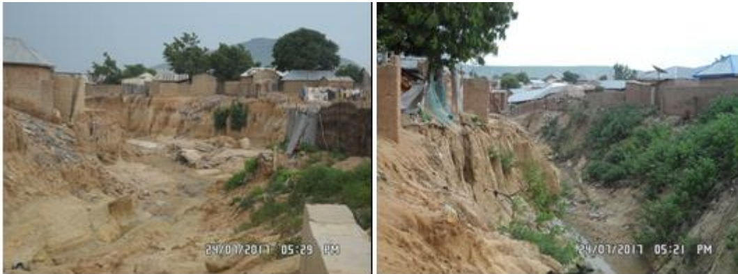
Plate 3: Gully channel outside the university campus (pindiga formation)
