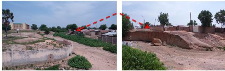
Plate 1: Eastern perimeter (cutoff) fence of the Gombe state university
