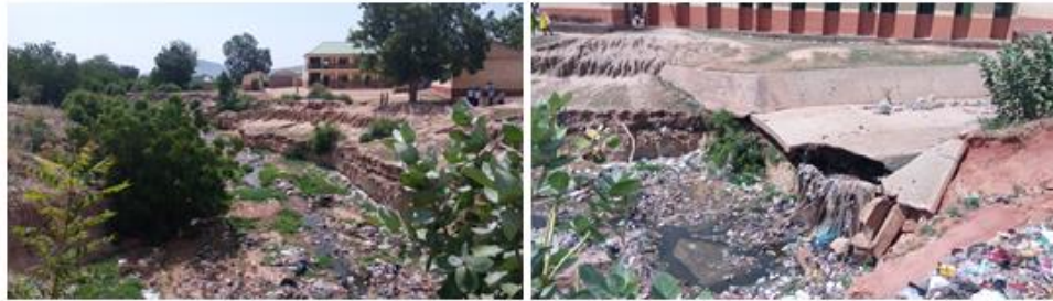
Plate 2: Gully channel in Gombe State University (left) termination of the gully project at the inlet (right).
