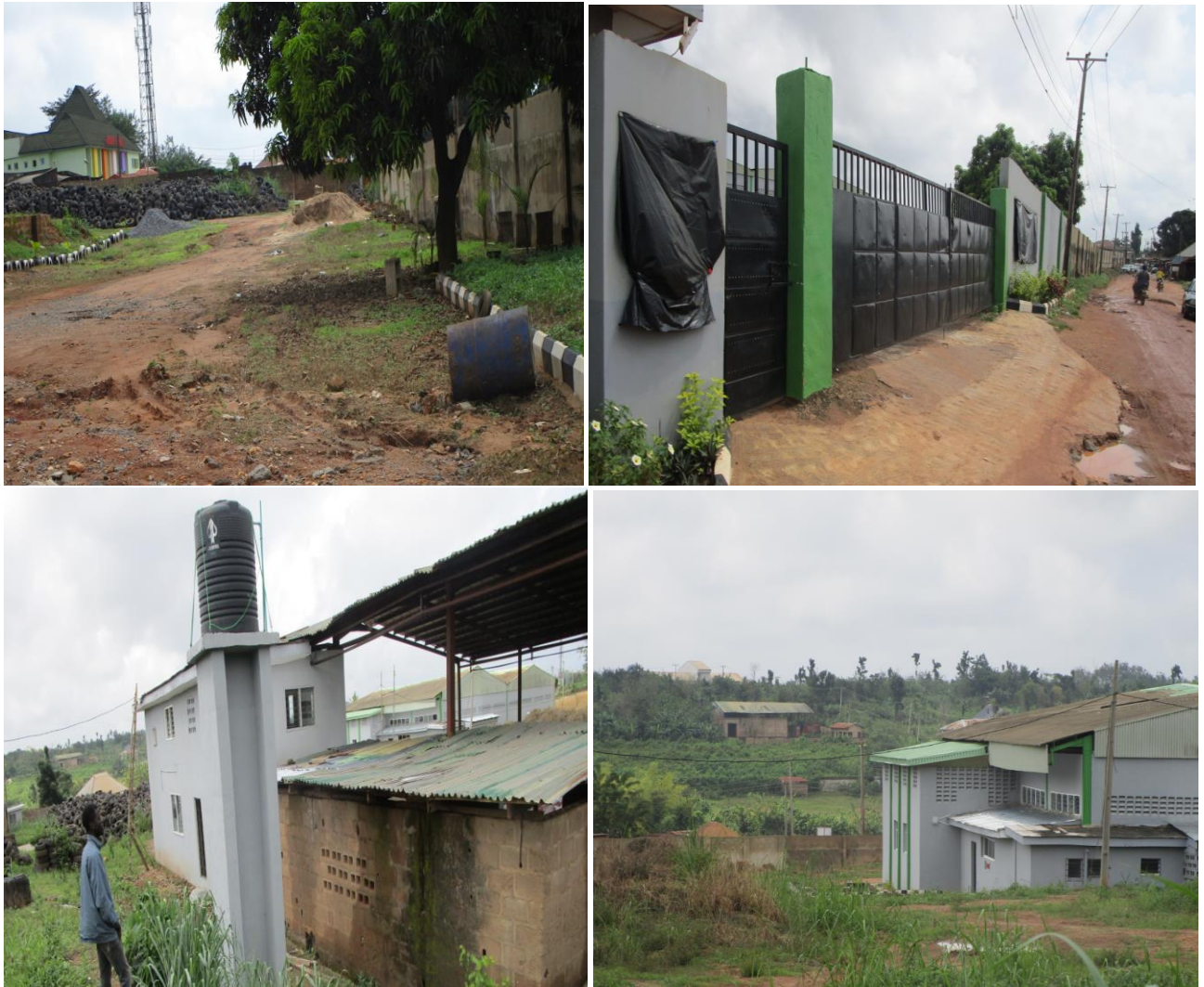
PLATE 4.5: PHYSICAL STRUCTURES WITHIN THE PROJECT LOCATION
