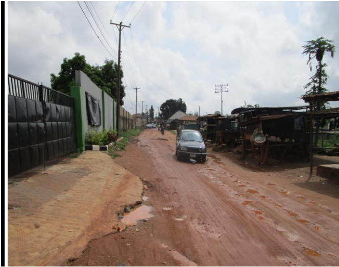
PLATE 4.10A: EARTH ROAD BY THE PROJECT SITE
