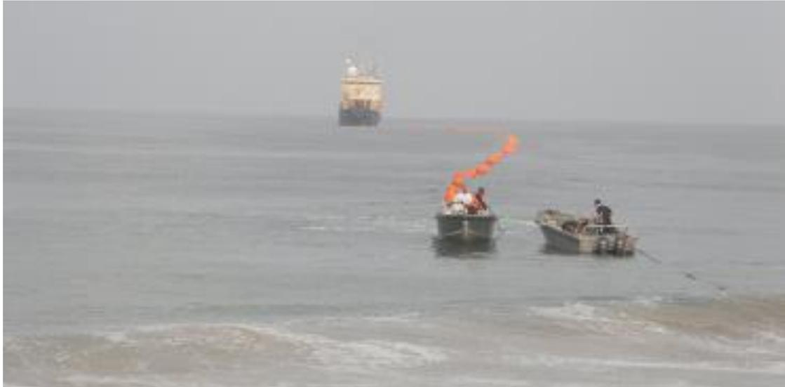
**Plate 3.5: Typical cable landing operation (ASN, 2020)**
