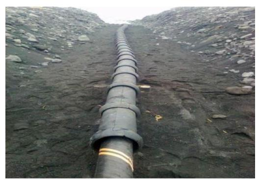
Plate 3.6: Typical articulated pipes installed on cable (ASN, 2019)
