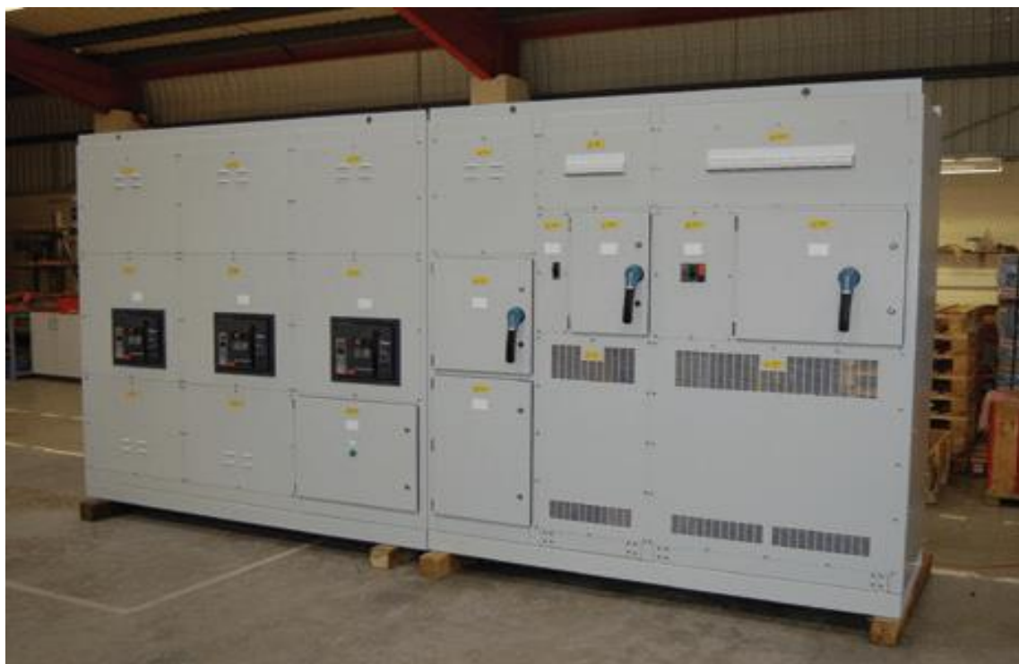
Plate 3.2: A typical low voltage switchgear cabinet
