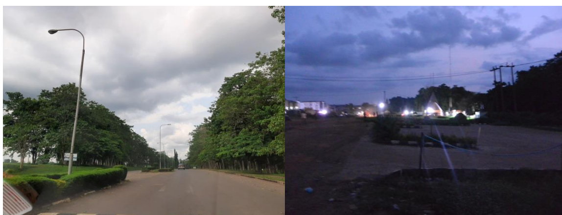
Plate 3.3: Sample of streetlights in FUNAAB campus
