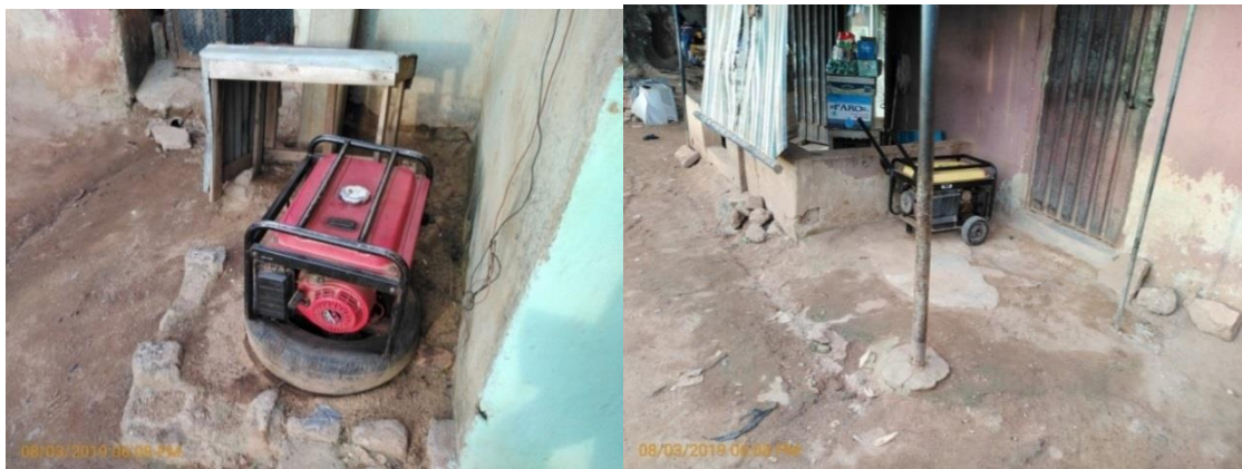
Plate 4.13: Generator as alternative source of electricity found in the village
