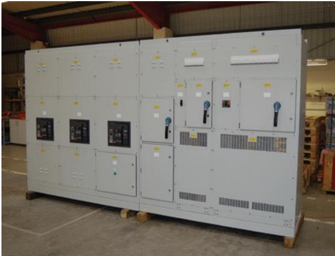
Plate 3.3: A typical low voltage switchgear cabinet
