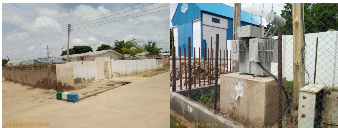
Plate 4.10: Electricity infrastructure observed in Low Cost Community
