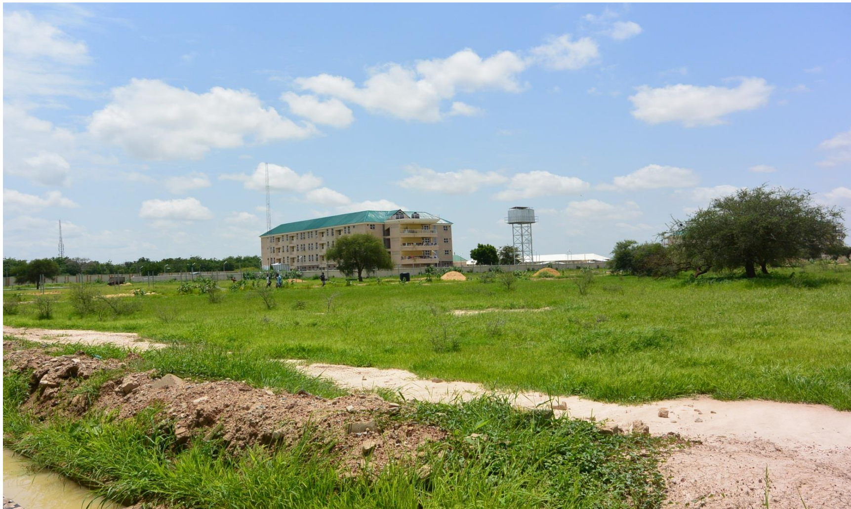
Plate 3.1: Cross-sectional view of the Project Site within FUGA campus (during the rainy season) (Source: EnvAccord fieldwork, 2019)
