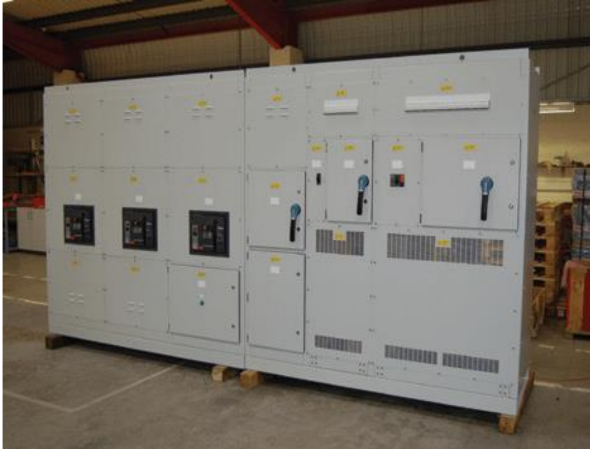
Plate 3.2: A typical low voltage switchgear cabinet
