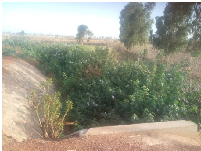
Figure 5: Drainage culvert with overgrown vegetation blocking water passage and causing flood in adjoining farmland
