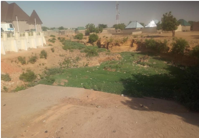
Figure 3: Part of the gully beside a fuel station which needs to be quickly addressed to prevent destruction
