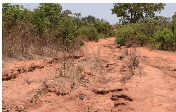
Plate 3.1: Failed and narrow portion at Mazakuka
