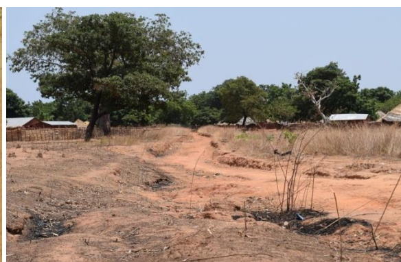
Plate 3.4: Failed portion along Mazakuka road
