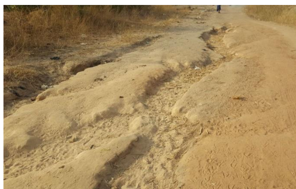
Plate 3.3: Failed portions at Daban
