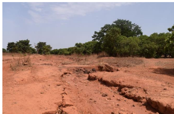
Plate 3.2: Failed section along Adogon-Mallam Road
