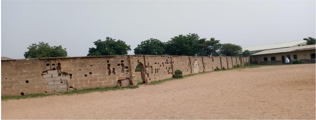
**Plate A.6:** Security fence breach
