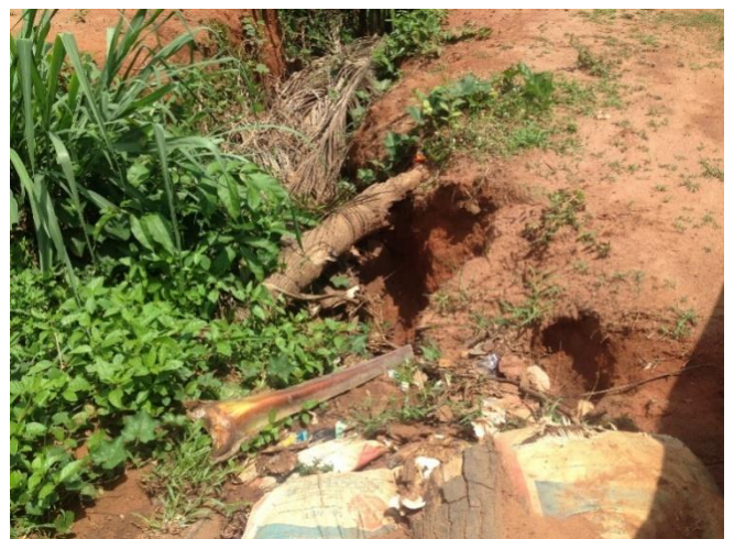
Plate 41 Sand Bags used to control erosion by community
