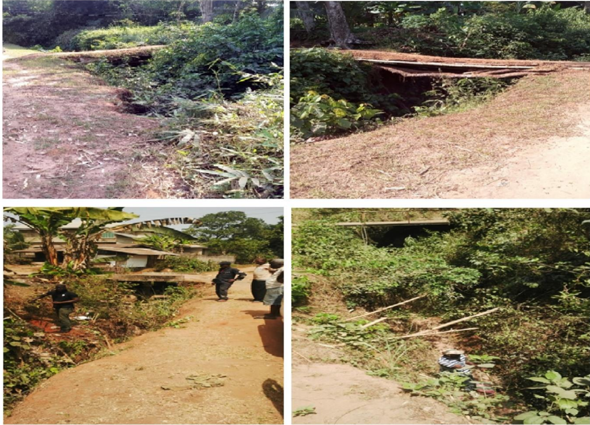
Fig. 7, 8, 9 & 10: Timber/Bamboo access bridges to people's houses
