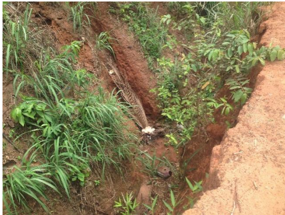
Plate 7: A section of the erosion
