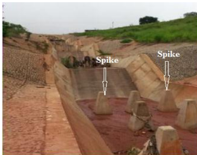
Plate 3.5: Stepped baffle chute
