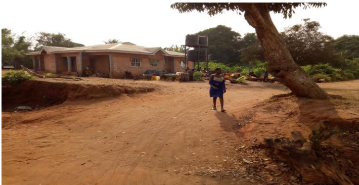
Plate 4.10: Private Borehole Water Providing Water for the Residents of Ewu Town
