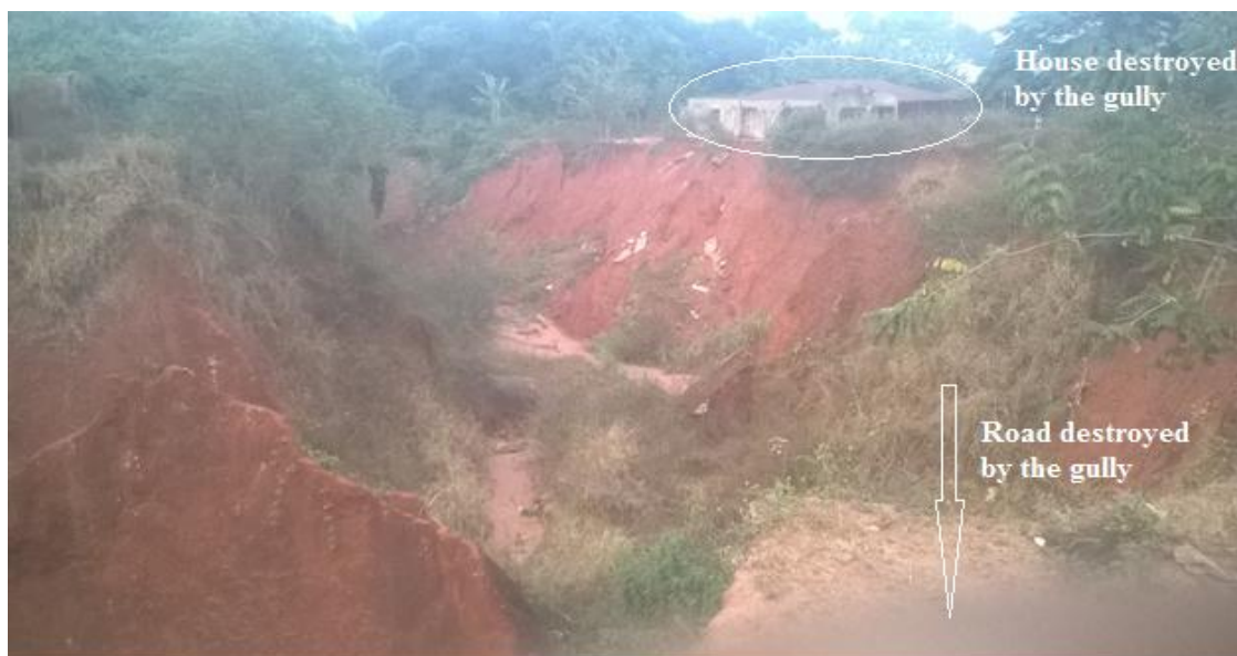
Plate 3.2: Gully at Ewu showing some affected Houses and Tarred Road as at March 2017
