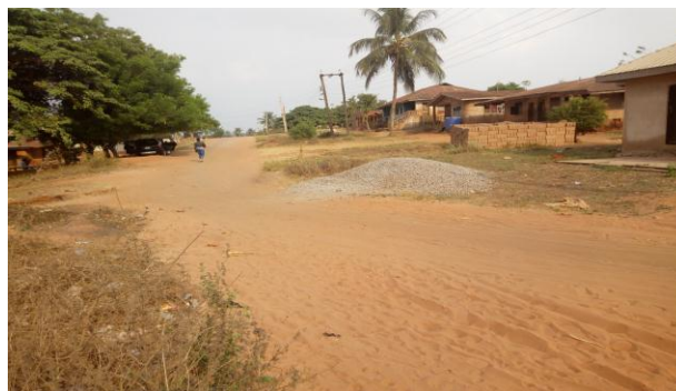
Plate 4.8: Low Tension Electricity Line in Ewu Town
