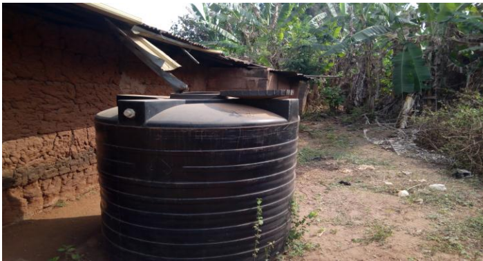
Plate 4.9: Rain Water Harvesting in Ewu Town
