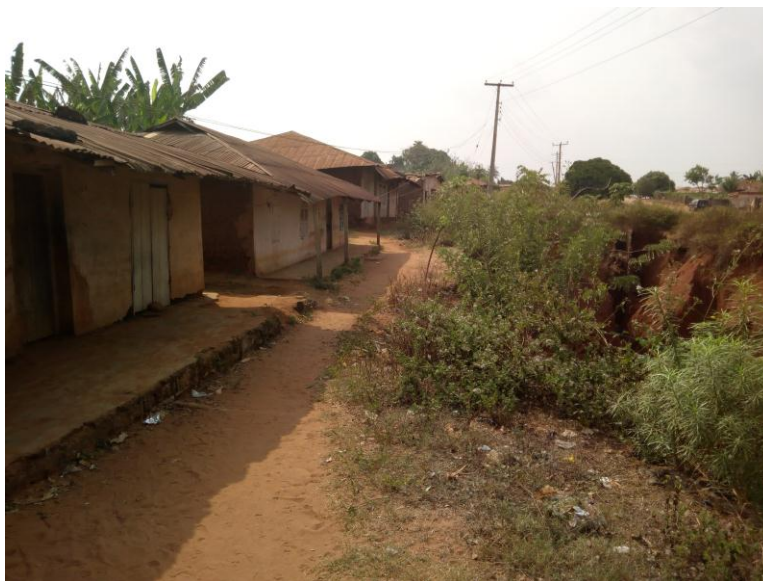
Plate 4.5: Semi-Detached Buildings in the Vicinity of the Gully Erosion Site
