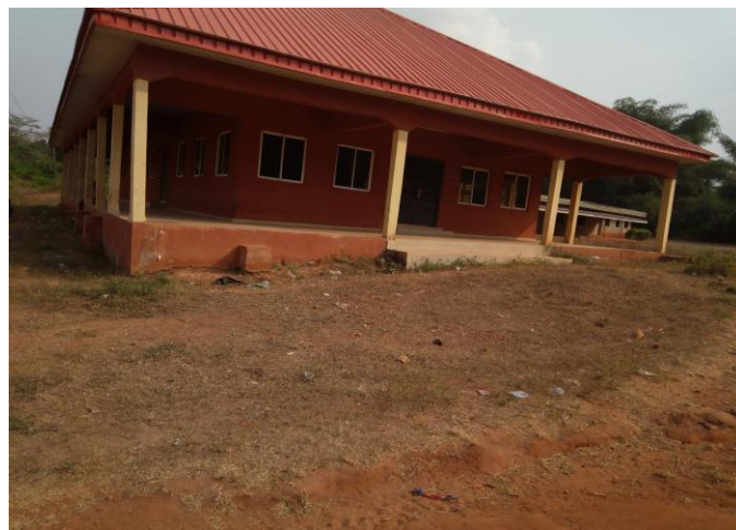
Plate 4.7: Long Span Aluminium Used in the Ewu Town Hall
