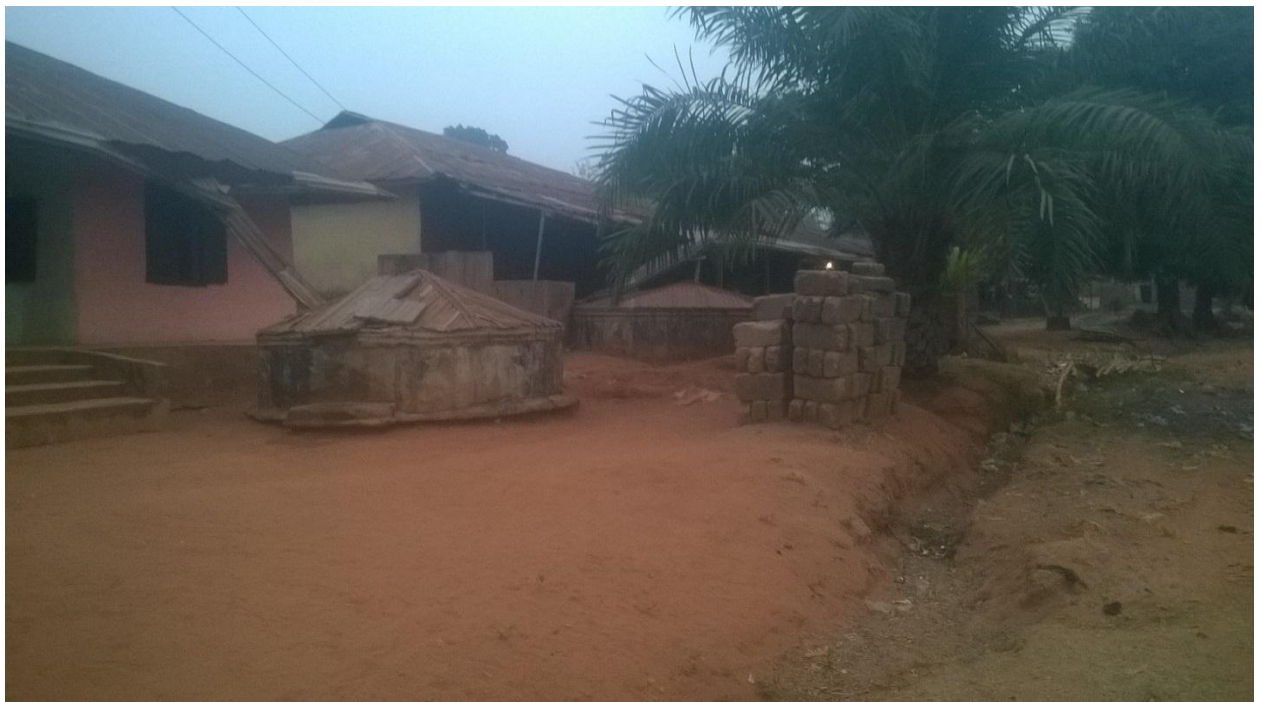
Plate 3.4: Typical Rainwater Harvest Facility at Ewu
