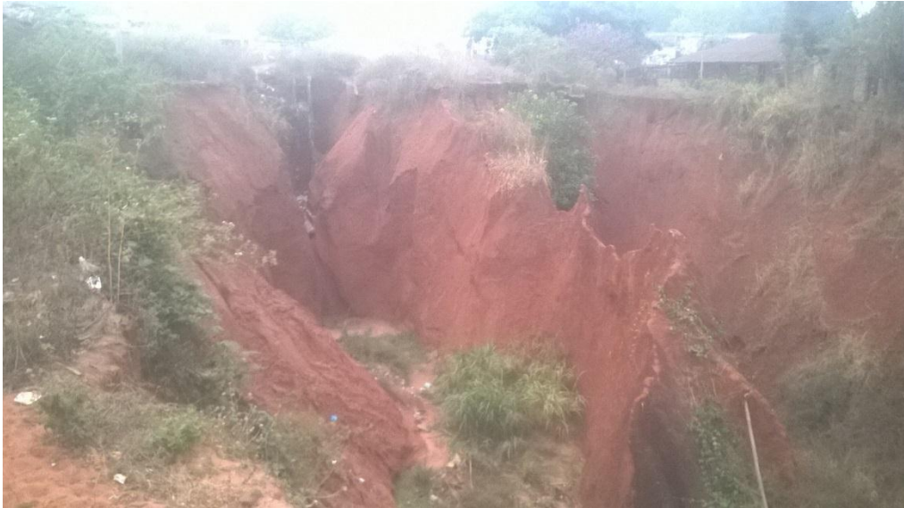
Plate 3.1. A section of the Gully in Ewu, Esan Local Government Area of Edo State, Nigeria
