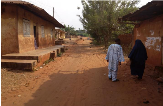
Plates 4.23: Eroded Building Foundation Consequent upon the Flood
