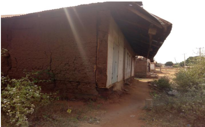
Plate 4.6: Mud and Block Materials Used in Building Construction in the Vicinity of the Gully Erosion Site
