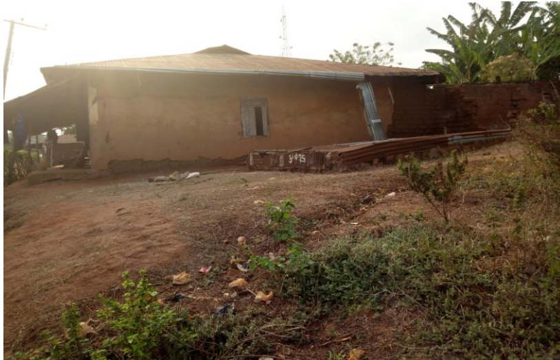
Plate 4.4: Rainwater Harvesting Device in Ibore Community
