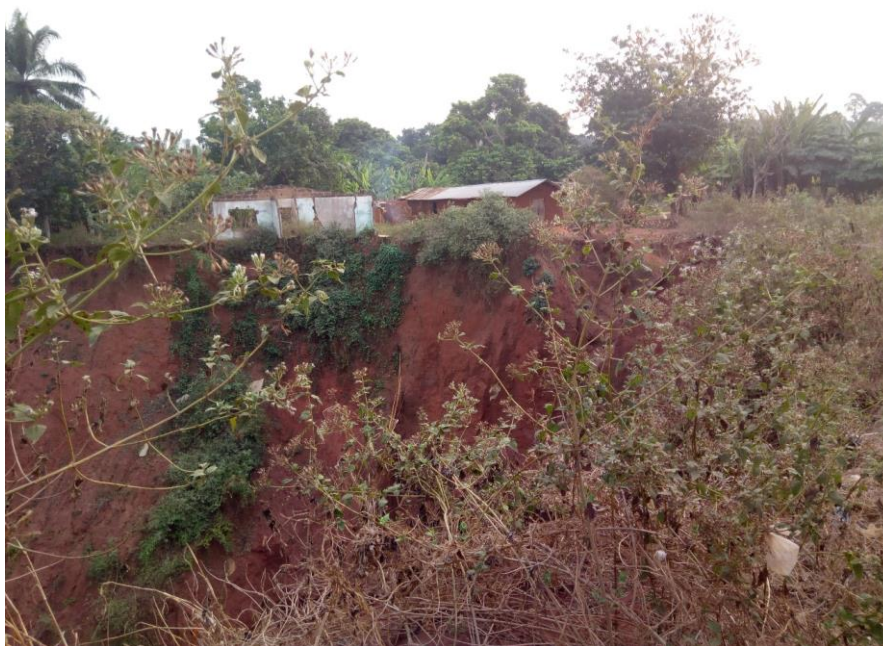
Plate 4.7: Building being threatening by the Expanding Gully in Ibore Community
