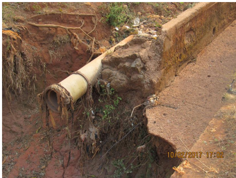
Plate 3.2: Gully at Ibore showing the broken stormwater pipeline that contributes to the gully erosion and the affected Tarred Road as at February 2017
