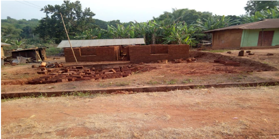
Plate 4.2: Typical Wall Materials Used in Building in the Ibore Community
