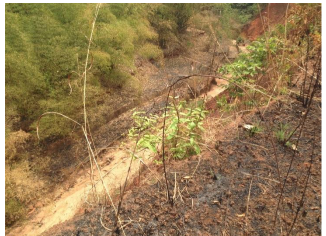
Plate 6 Concrete canal constructed by the community to control further erosion.
