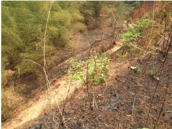
Plate 49 Canal built by community to check erosion
