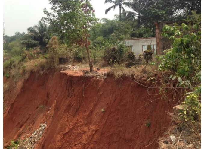
Plate 4 A section of the Main Gully
