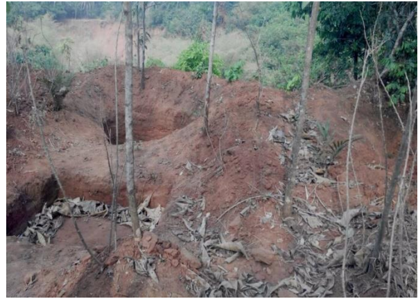
Plate 48 Catchpit dug by community to check flooding
