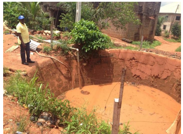
Figure 11 Catch pit constructed by residents
