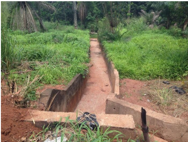
Figure 14 Drainage constructed to channel runoff at St. Theresa gully finger
