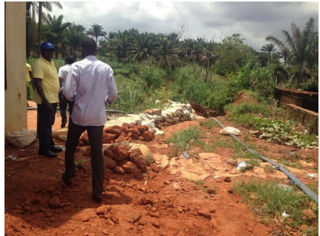
Figure 9 sand bags used by residents to check the gully
