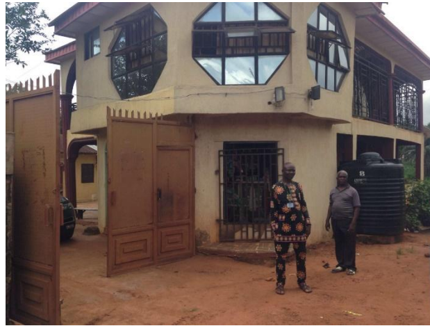
Figure 12 Building threatened by the gully
