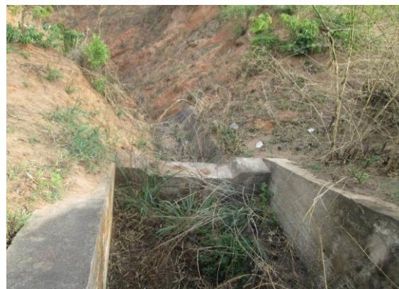
Plate 1.2: Existing trapezoidal channel
