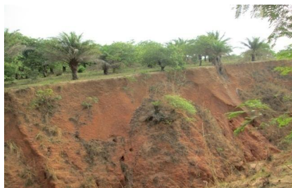
Plate 1.4: Farmlands destroyed by the Gully
