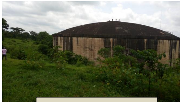
Ground level reservoir
