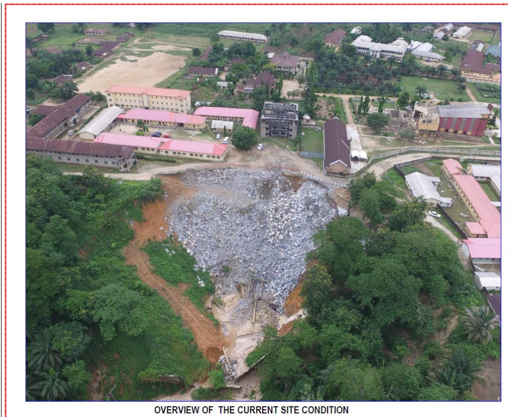
Plate 3.1: St. Luke's hospital, Anua Gully Erosion Area of Influence
