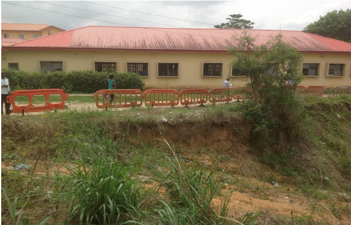
Plate 3.6: Earth road and buildings at risk of collapsing
