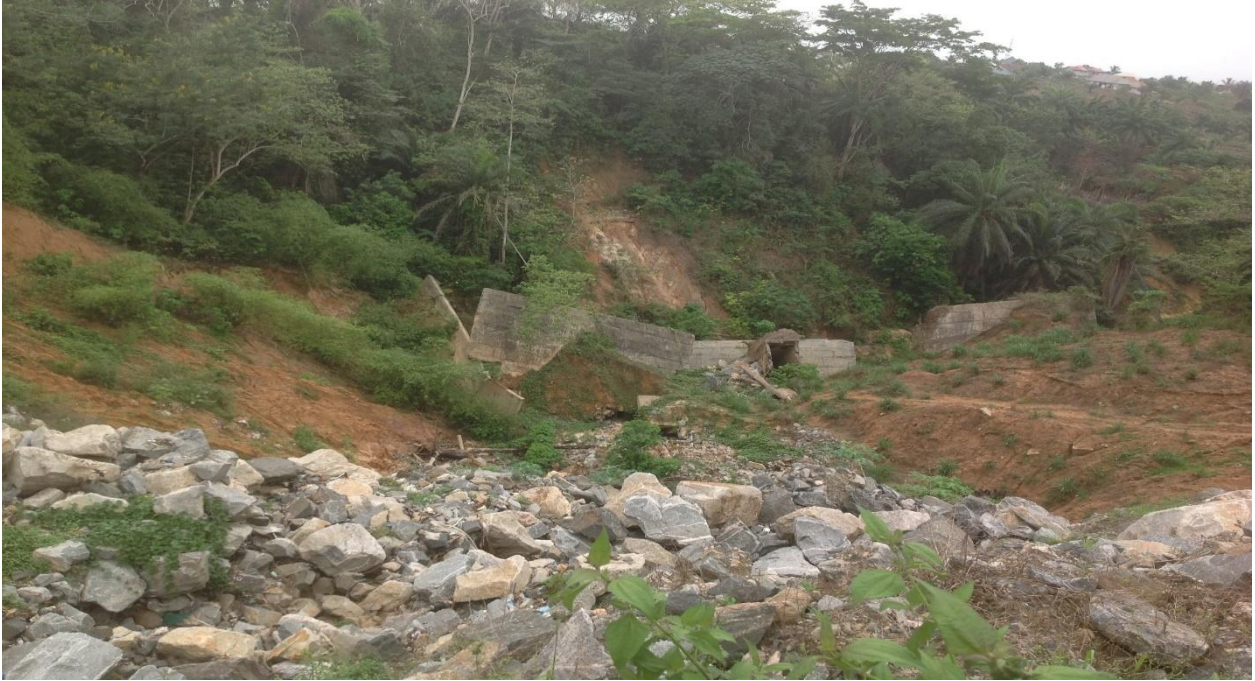
Plate 2.2: Anua Offot Gully Erosion Site- Uyo L.G.A
