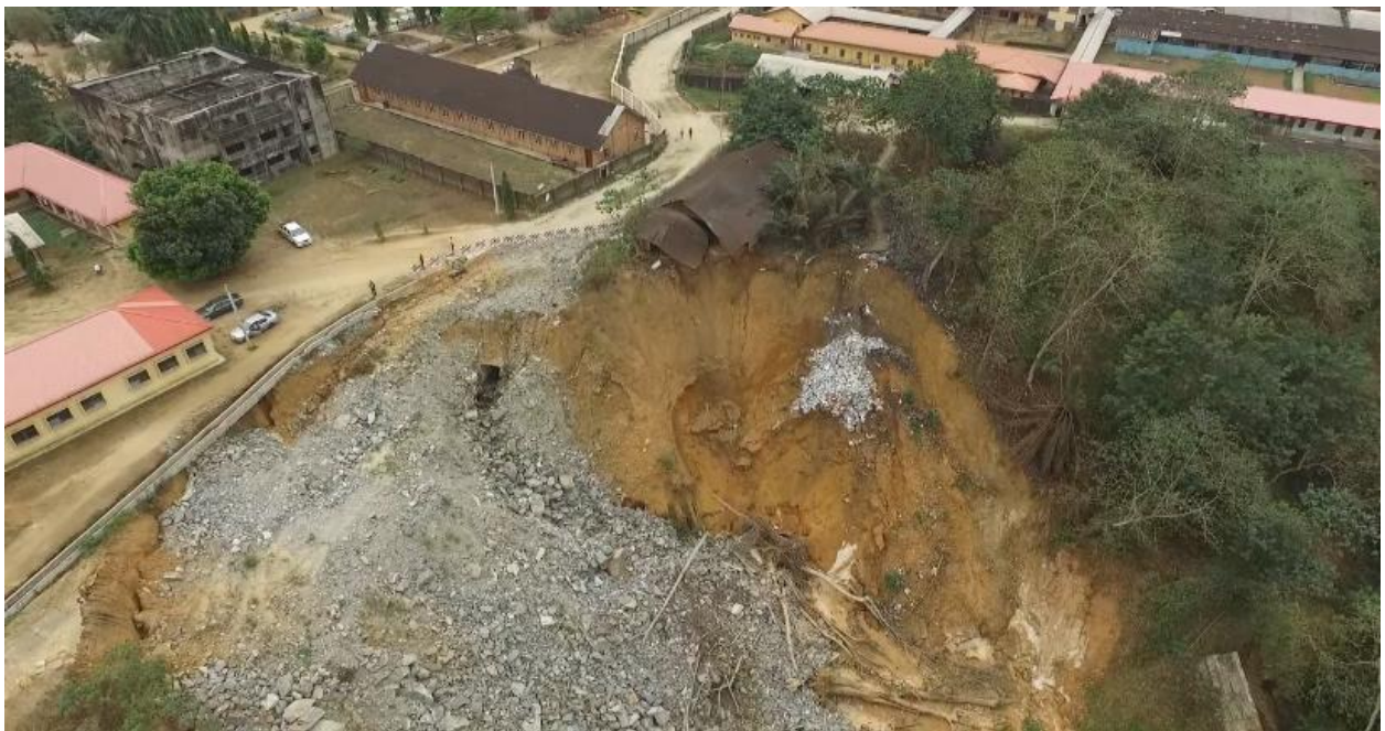
Plate 2.1: Anua Offot Gully Erosion Site- Uyo L.G.A.
