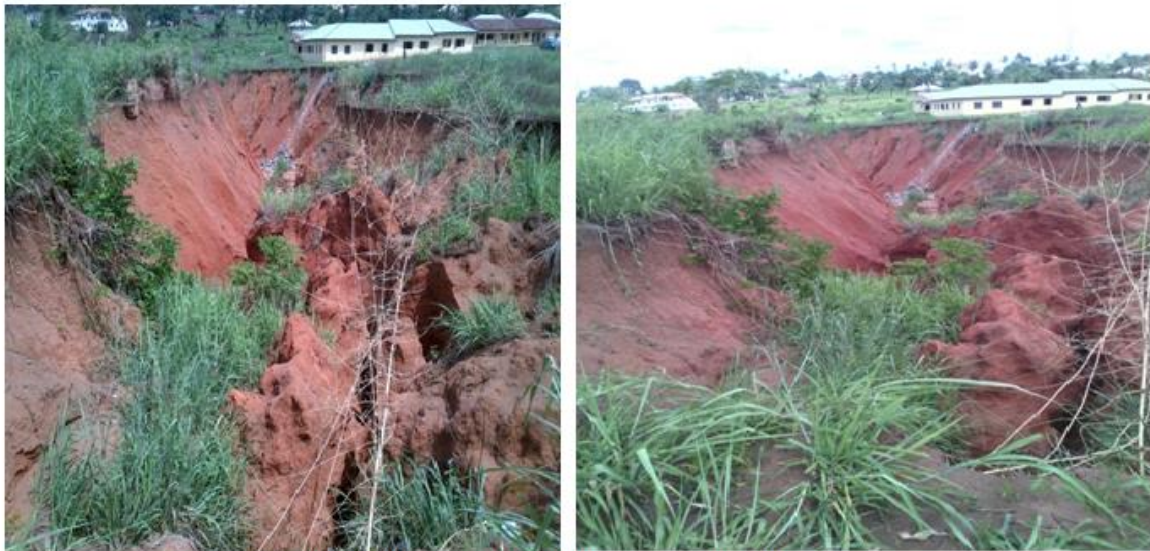
Fig. 4 & 5: Umuagu primary school buildings under threat of the gully
