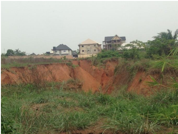
Plate 7 A section of the gully with a threatened building
