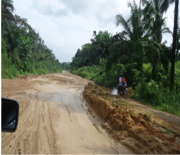
Plate 27: Delapidated Calabar-Bakassi Road in Atignbo community
