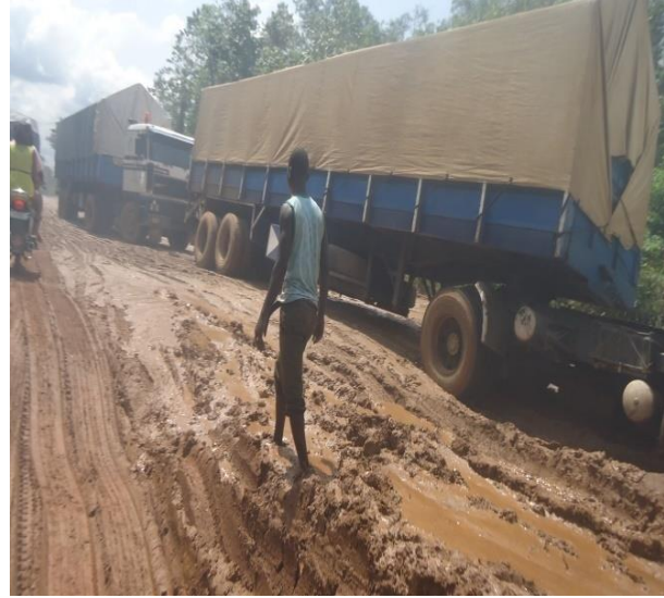
Plate 28: A Failed portion of the existing Ikom-Calabar Road in Obubara community
