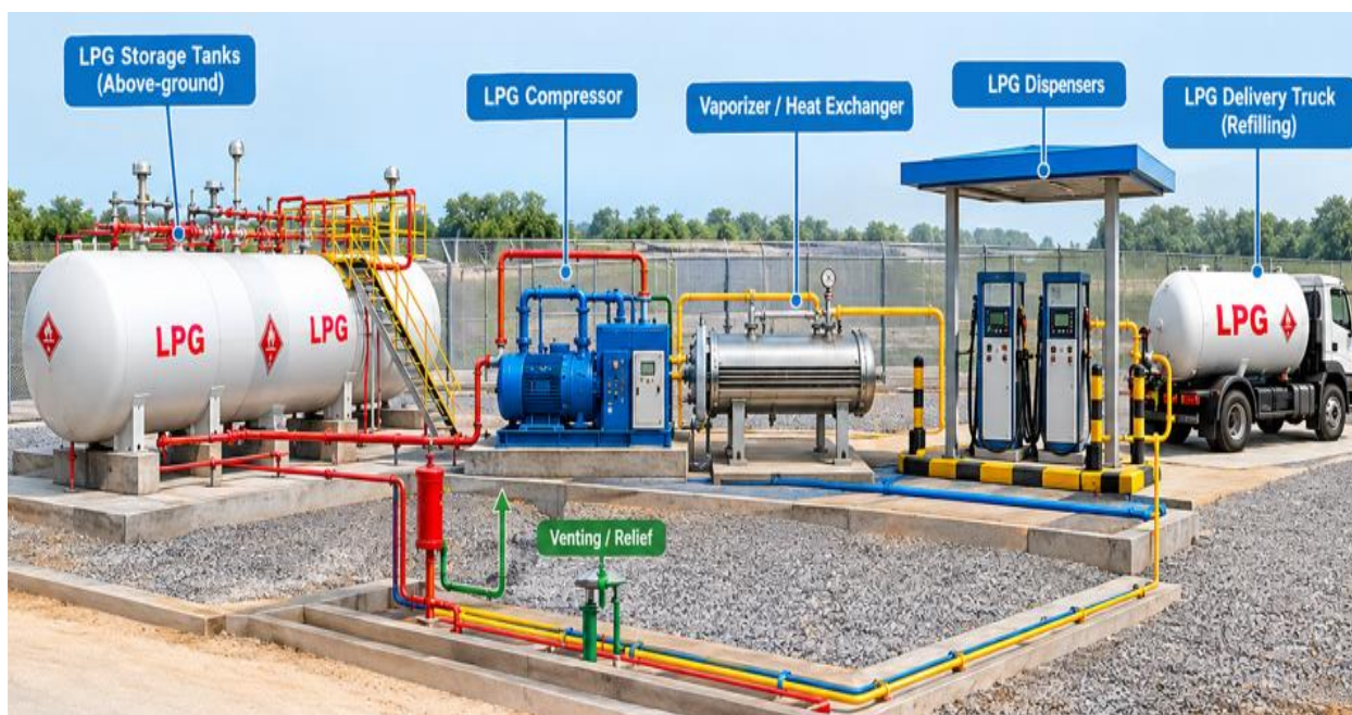
Figure 3.3: LPG Storage, Compression and Dispensing Process
