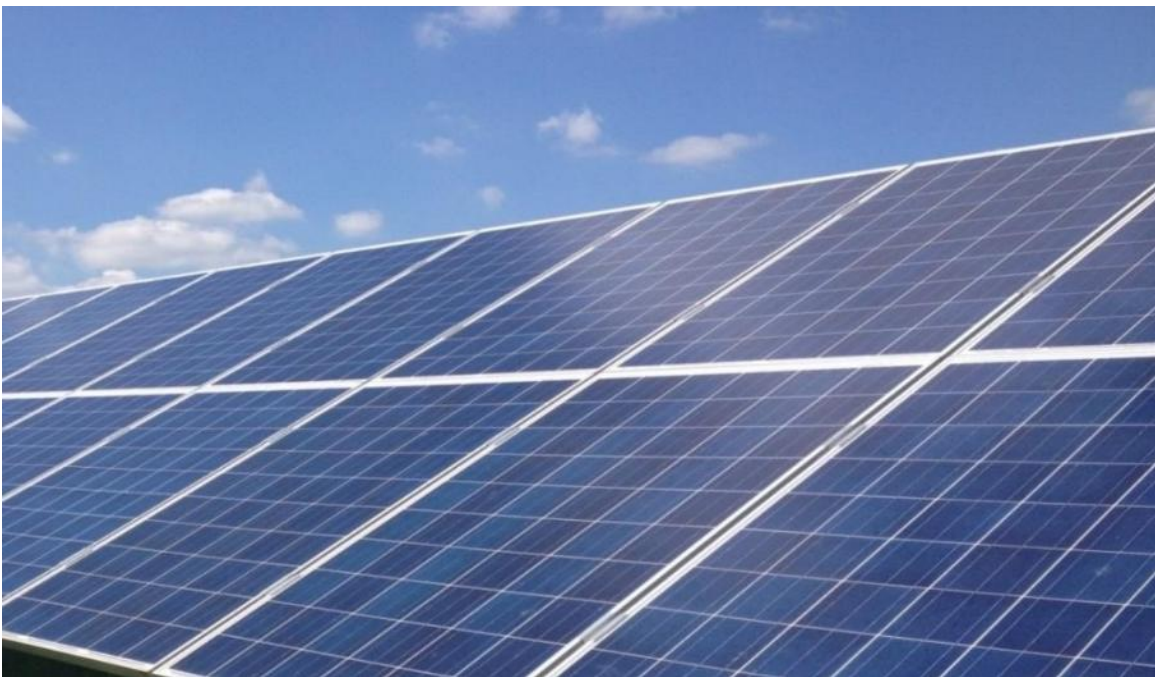
Plate 2.2: Typical Appearance of Polycrystalline Silicon PV panels
