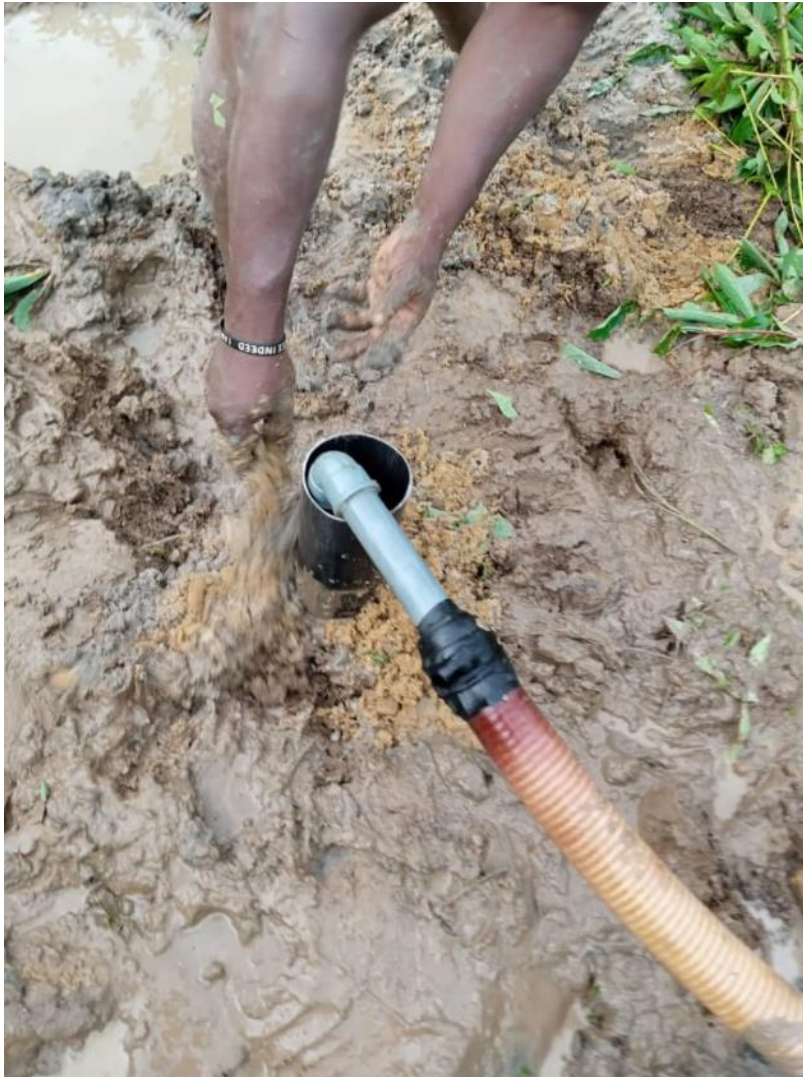
Plate A2: Borehole monitoring well (ongoing drilling)
