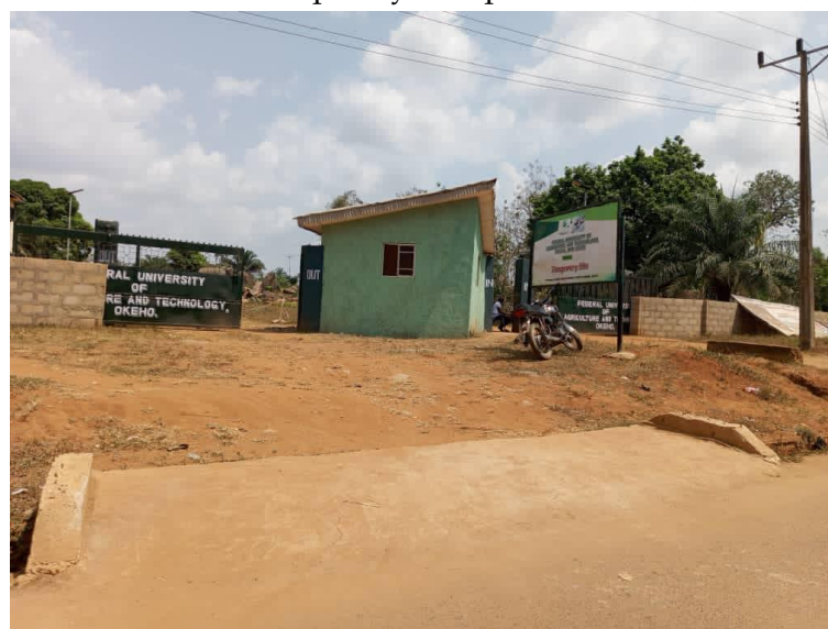
Plate 4. 3: FUNATO Temporary Campus Main Gate, Okeho, Oyo State
