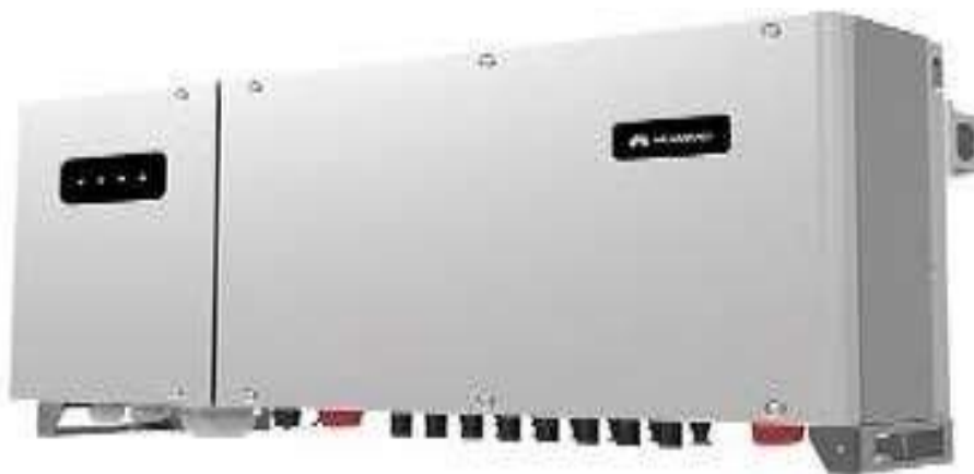
Figure 3.3: Example of string photovoltaic inverter (Source: REA Desert to Power Initiative (Phase II) FEED)
