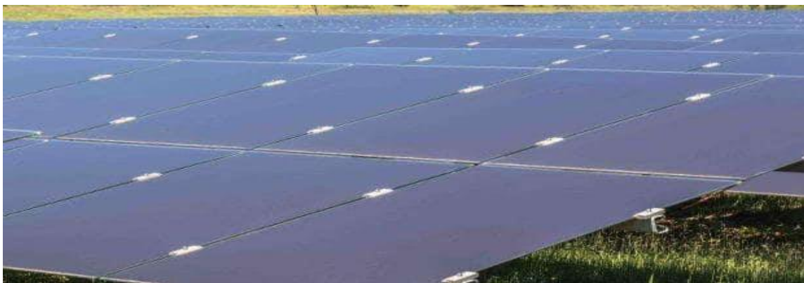
Figure 2.4: Typical appearance of Thin-Film CdTe panels
