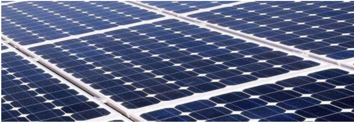
Figure 2.2: Typical appearance of mono-crystalline silicon PV panels
