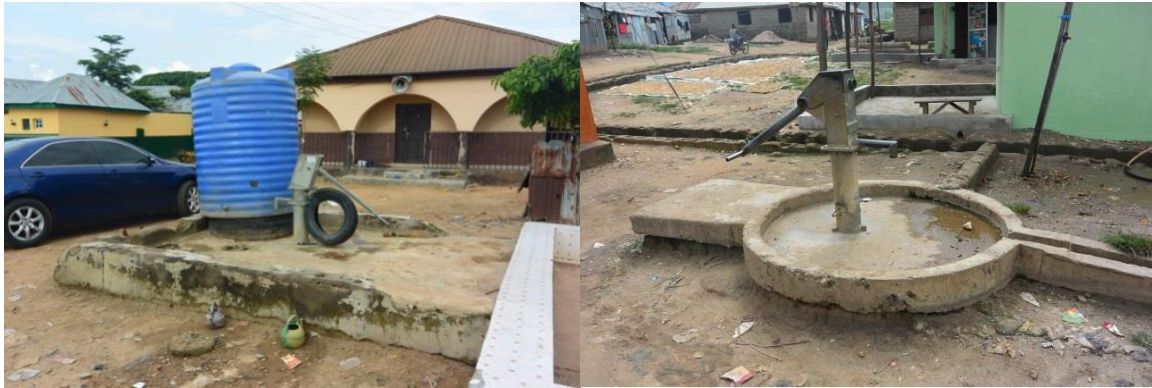
Plate 4.18: Water facilities found within the community
