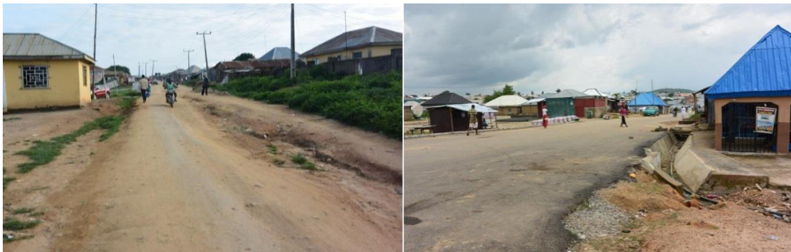
Plate 4.20: Road networks linking into the main community
