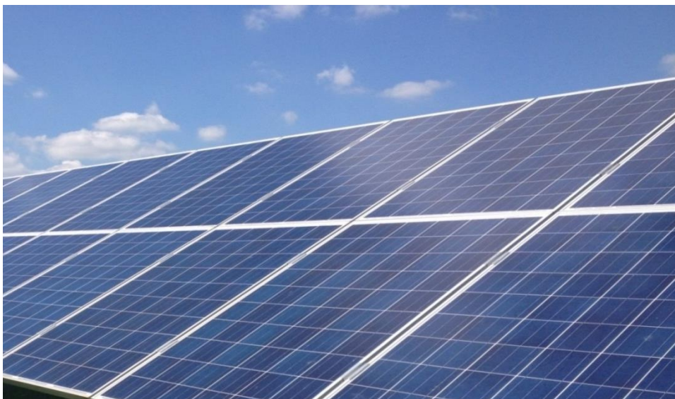
Figure 2.3: Typical Appearance of Polycrystalline Silicon PV panels
