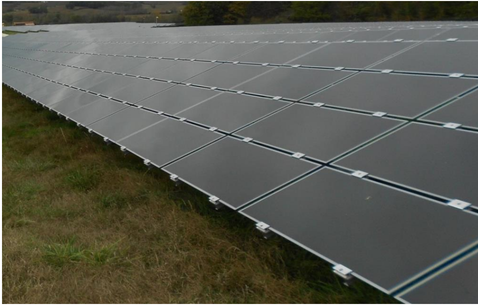
Figure 2.4: Typical appearance of Thin-Film CdTe panels
