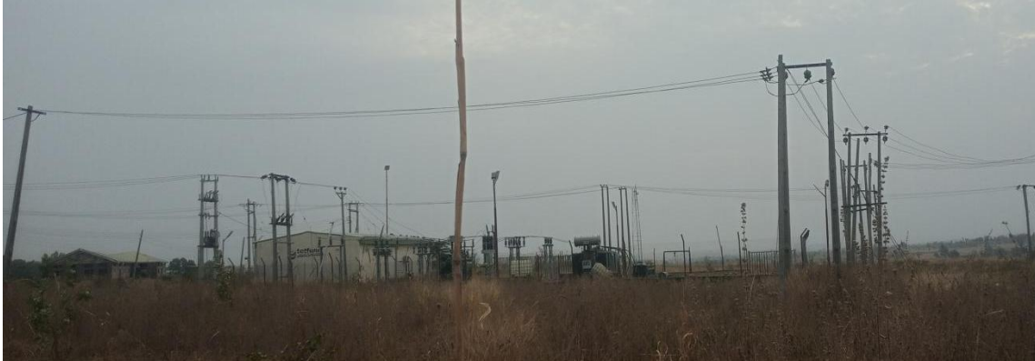
Plate 3.7: Showing an existing electric distribution infrastructure situated beside the proposed project site (existing electric sub-station of FUT Minna)
