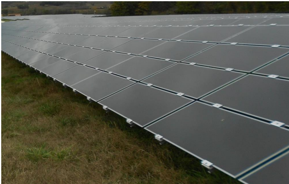
Figure 2.4: Typical appearance of Thin-Film CdTe panels
