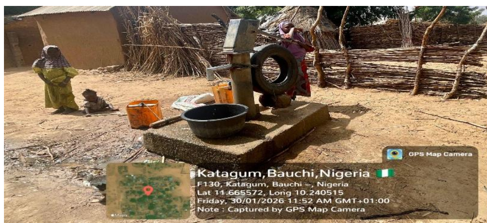
Plate 4.15: Mechanical Hand Pump Borehole in the project AoI
