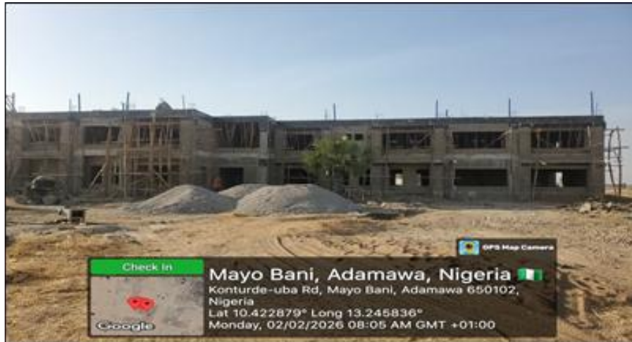
Figure 4: Ongoing Construction Activities at the Broader Premises of the Project Site.
