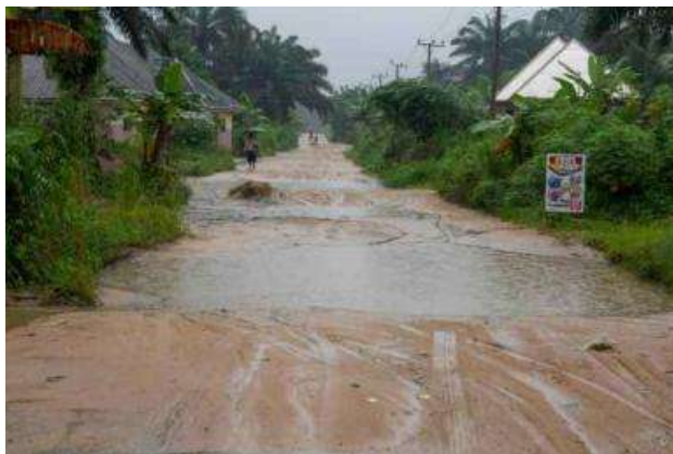
Appendix I.2: Community access road during wet season (April 2026) — severe flooding of laterite road surface illustrating baseline drainage and infrastructure deficit; confirms need for Axle Load Management Plan during construction
