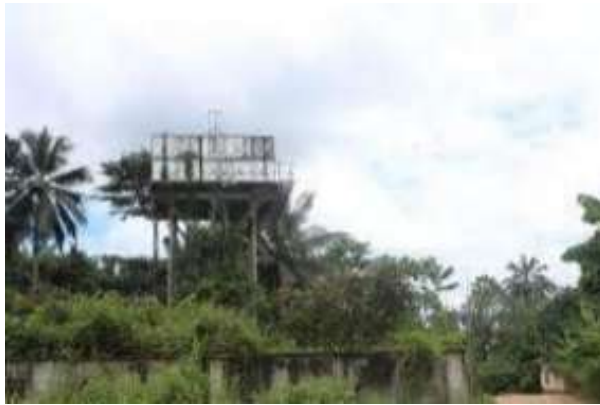
Appendix I.1: Community overhead water storage tank — Ikot Obio Offiong (baseline water supply infrastructure; confirms community reliance on elevated storage tanks and private boreholes rather than piped supply)
