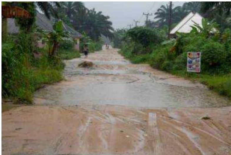
Plate 4.3: Community access road during wet season — flooded laterite road illustrating existing drainage and infrastructure deficit
