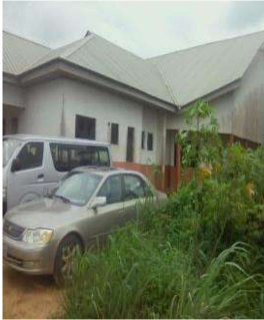
Appendix I.4: Typical community housing stock — block construction with corrugated iron roofing, partially developed compound (baseline documentation, April 2026; confirms 70% 'fairly good' rating from PERA household survey)
