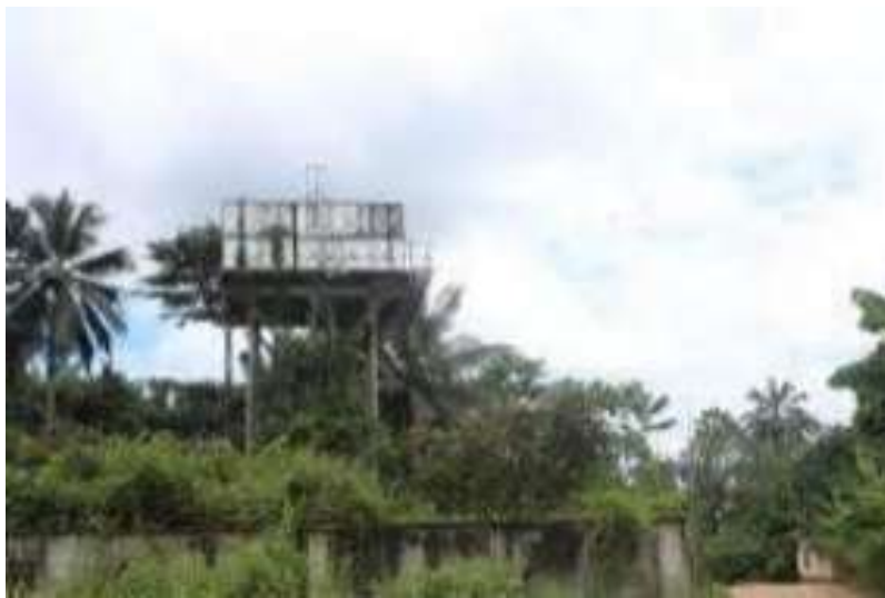
Plate 4.2 Community overhead water storage tank — Ikot Obio Offiong (baseline water supply infrastructure)
