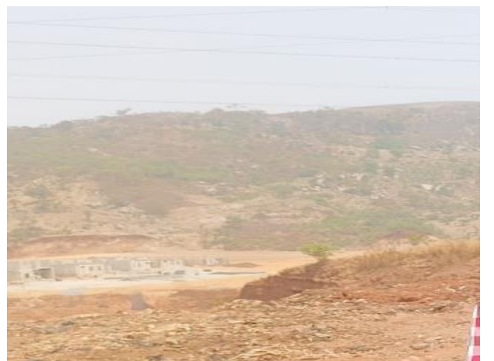
Plate 3.4: Undeveloped TCN High Tension Set-Back
