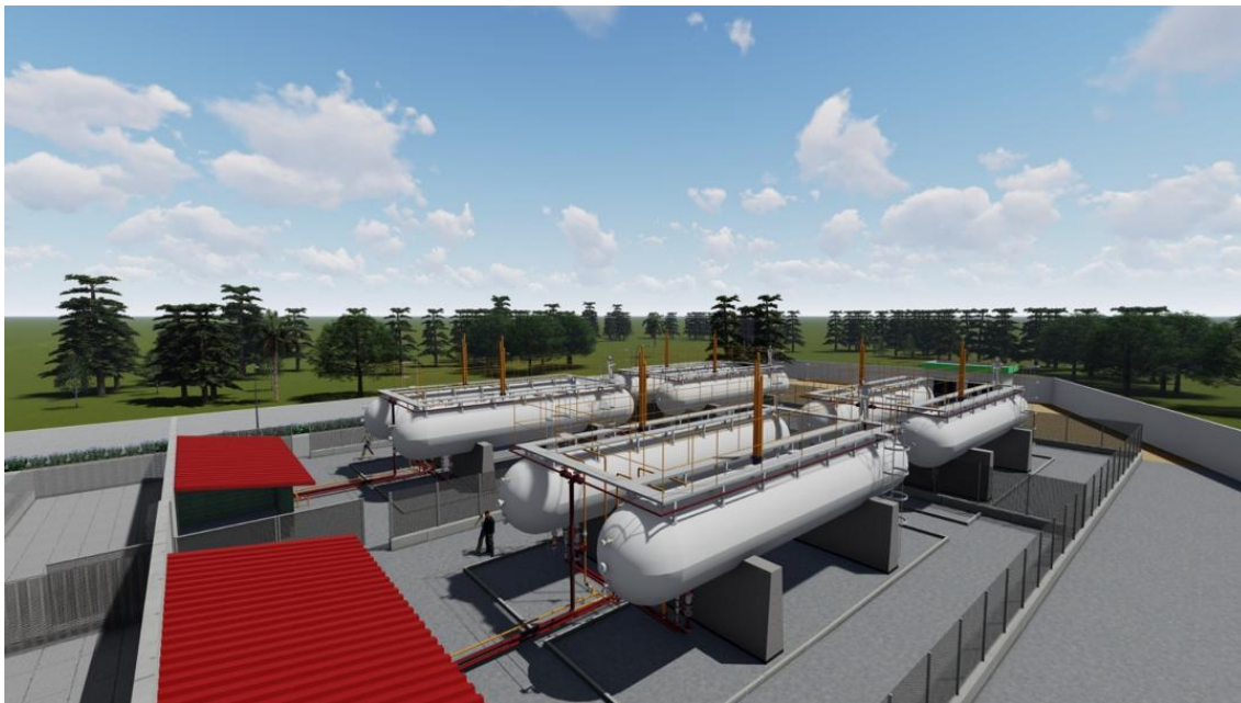
Figure 3.3: Storage System of LPG
