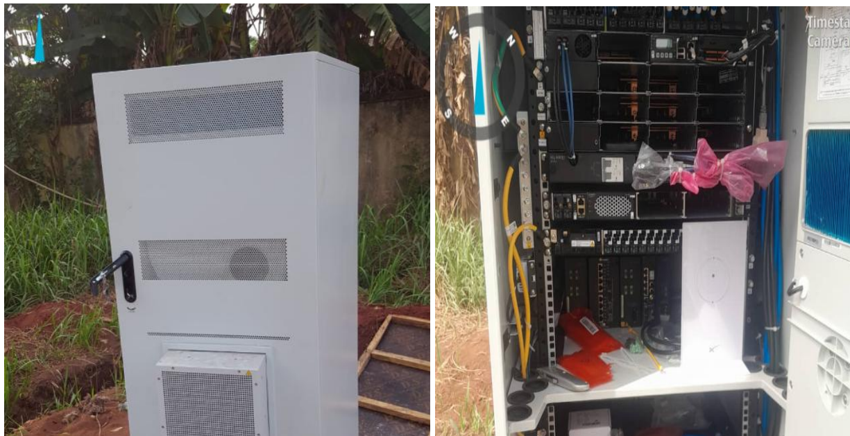
Figure 3.9: Wireless Network Rollout
