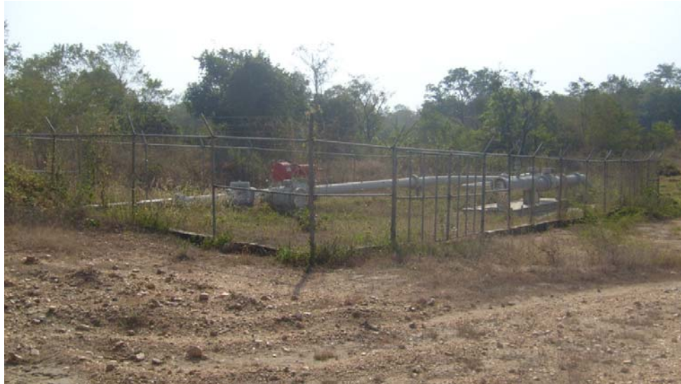
Plate 3.1: Ajaokuta Tie-in area
