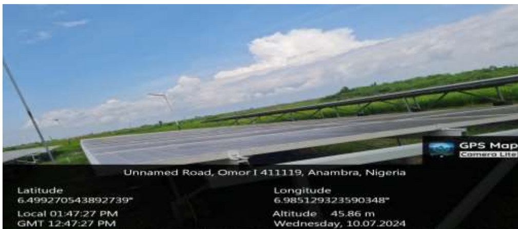
Plate 4.19: Solar farm project in Omor town
