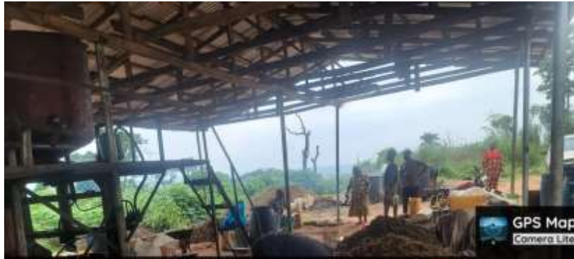
Plate 4.16: Small-Scale Oil Palm Processing Facility in Ogboji
