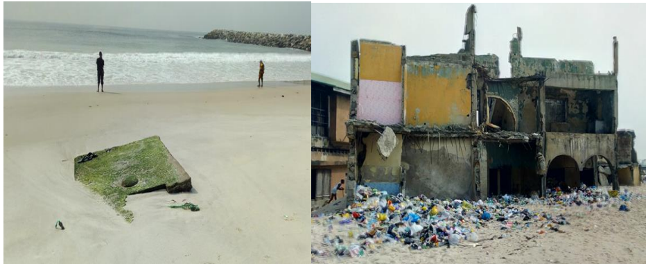
Plate 4.6: Submerged and damaged building at Alfa Beach, Eti Osa LGA
