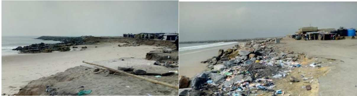
Plate 4.7: Failed access road in Alfa beach, Eti-Osa LGA
