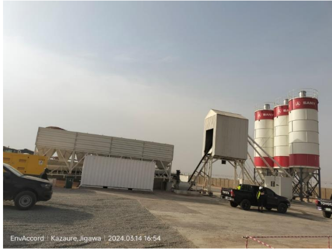
Photograph 37: Batching plant at Kazaure camp
