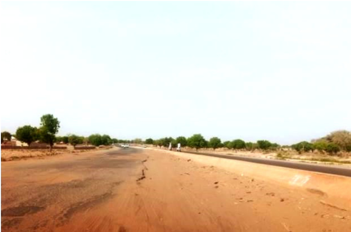
Plate 4. 11: A section of Kano to Dutse Road
