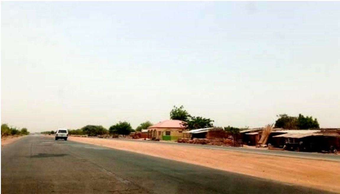
Plate 4. 13: A section of Kano – Katsina road
