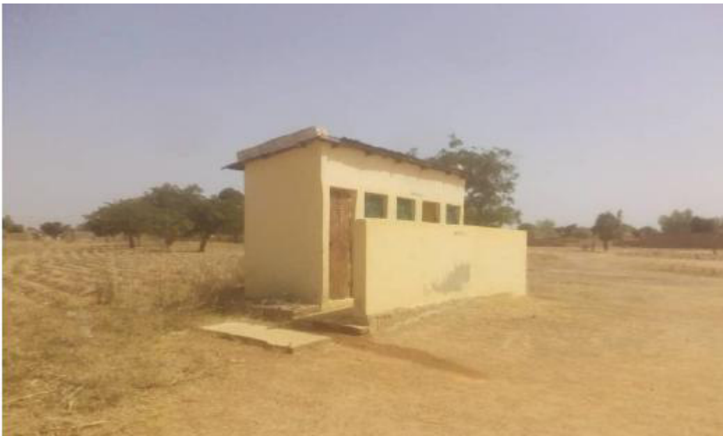
Plate 4. 44: Public toilet in Yumfuwa, Dawakin Tofa LGA, Kano State
