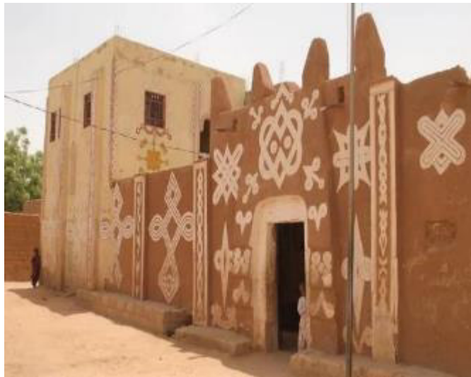
Plate 4. 46: Traditional Hausa Urban Architecture
