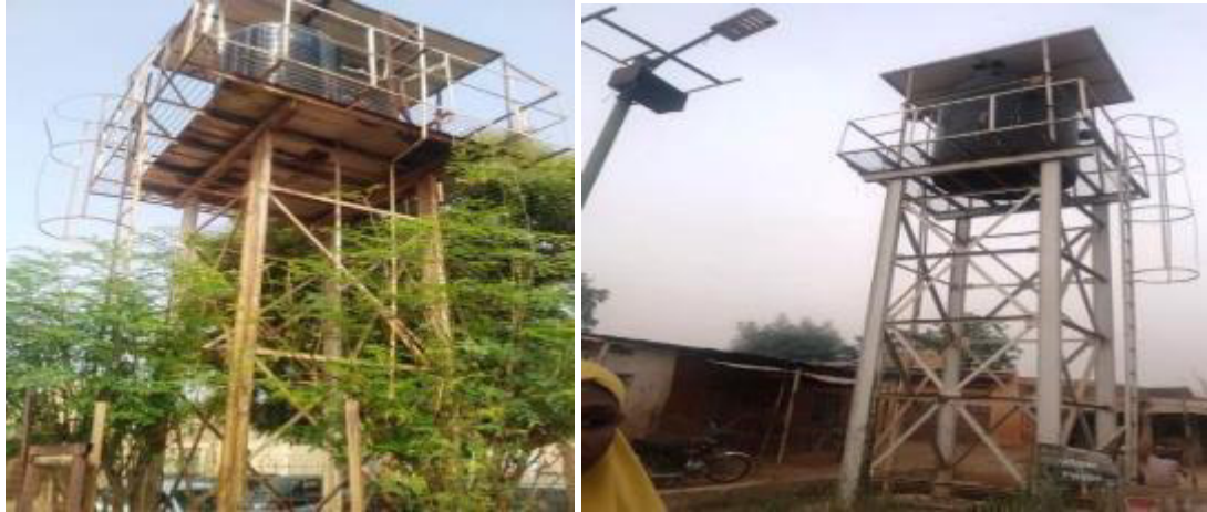
Plate 4. 41: Solar-powered Water facilities at Danbatta and Gwarabjawa
