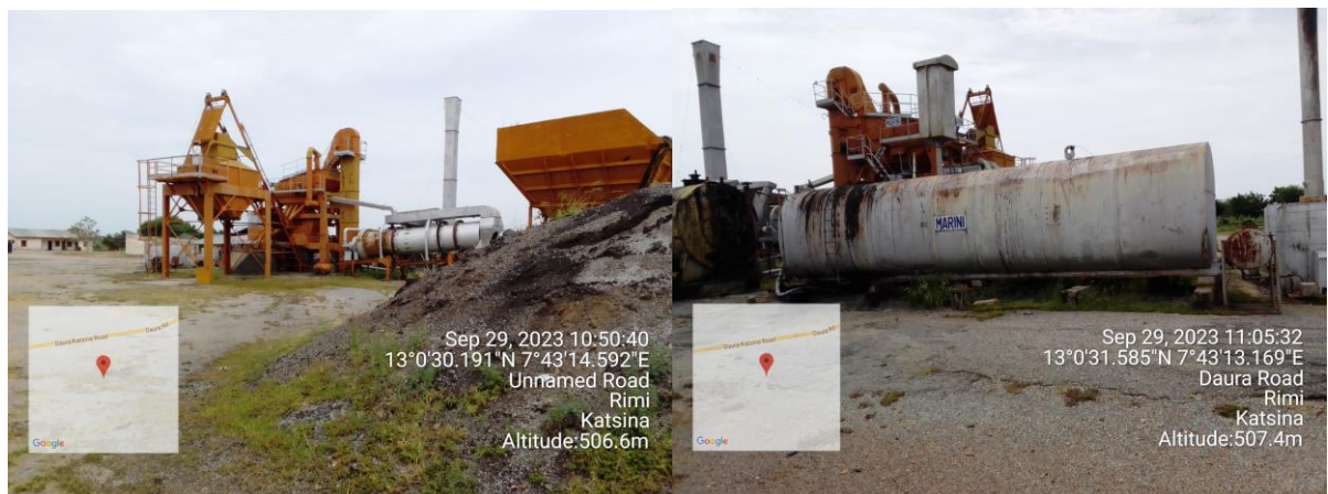
Plate 3.2: Abandoned Equipment within the Site (Snafhcore Limited Fieldwork September 2023)
