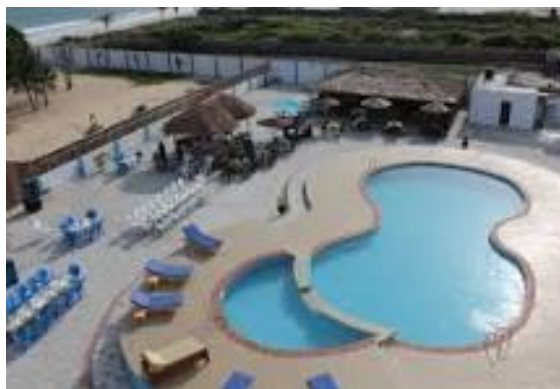
Plate 4.16a: Aerial View of Atican Beach Resort
