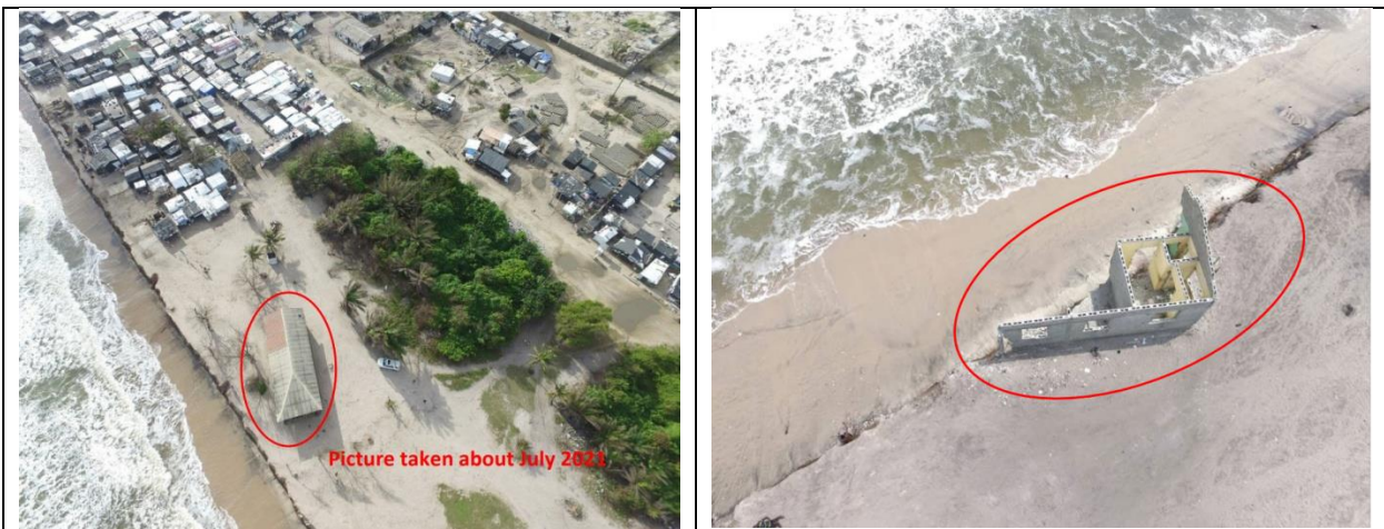
Plate 4.8: Coastal erosion along the Lafiagi – Alpha Beach axis
