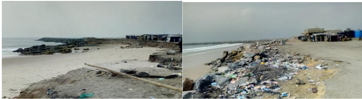
Plate 4.10: Failed access road in Alfa beach, Eti-Osa LGA
