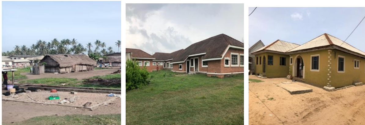
Plate 4.20: Roofing materials in the project area
