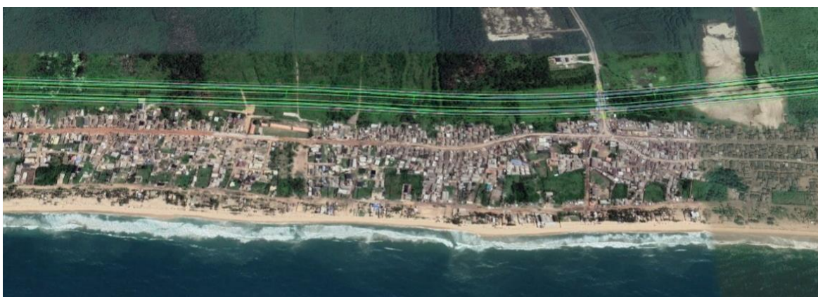
Plate 4.2: Satellite image of the proximity of buildings to the proposed road at Eleko village
