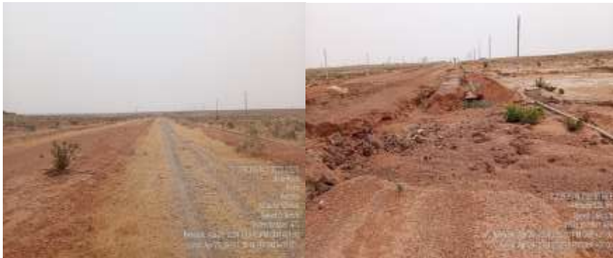
Sections of road under construction
