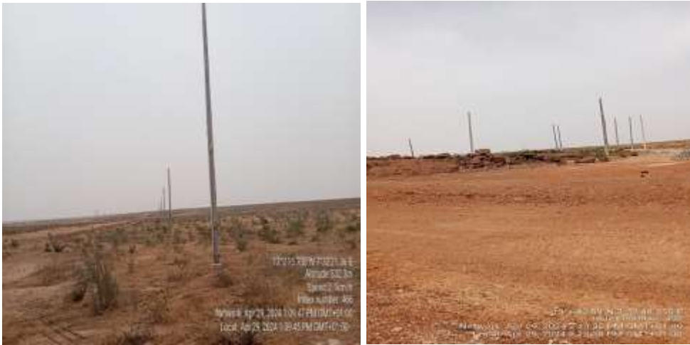
Electricity Pole installation
