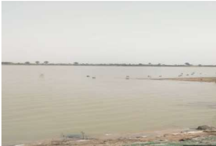
Parts of Doberam dam
