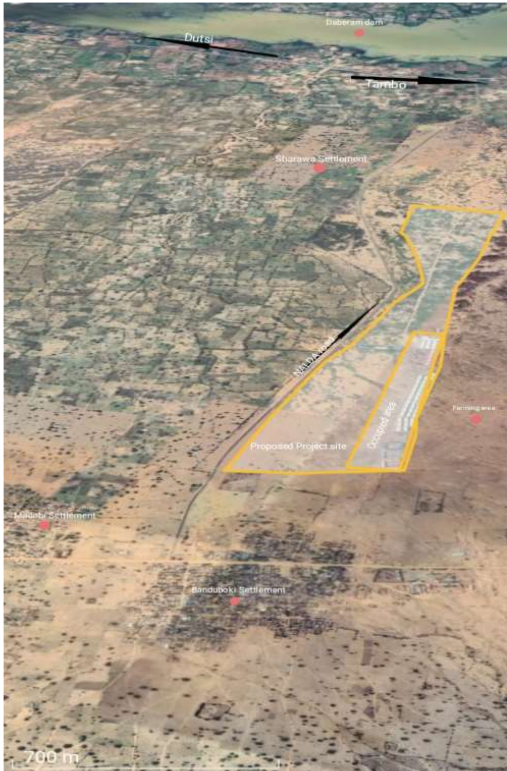
Figure 3.10: Google earth imagery of the proposed project site
