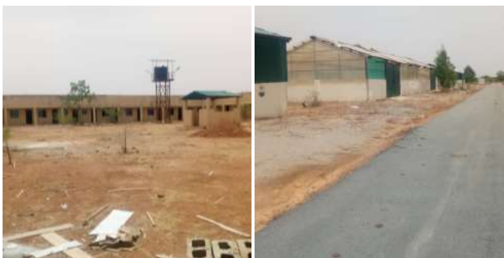
Infrastructures within the project site: Administrative building; Office blocks; Farm house
