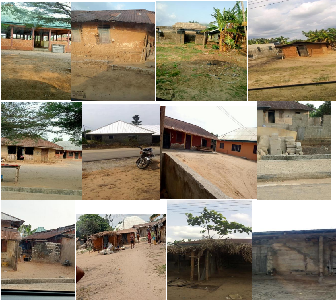
Plate 4.20: Roofing materials in the project area
