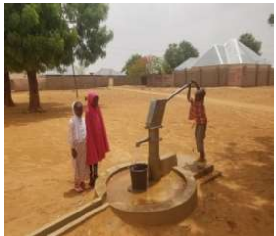
hand pump borehole
