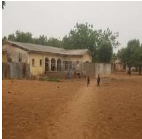
BSADP Staff quarters at the project site
