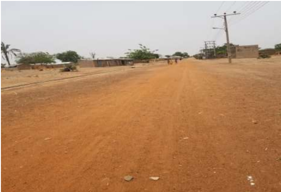
Plate 1.24: Untared road with drainage, connecting Malmo and Kuhu community.
