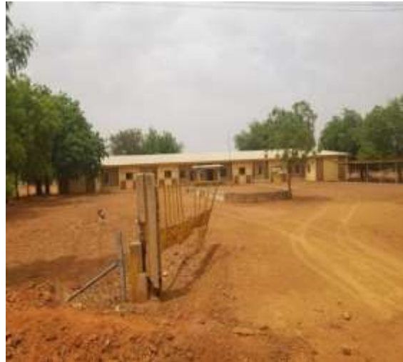
BSADP administrative building
