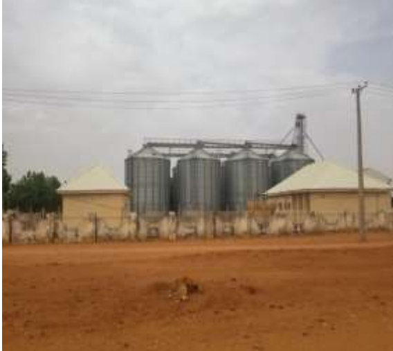
4000 tons food Silo at the project site
