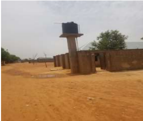
Water tank at the project site
