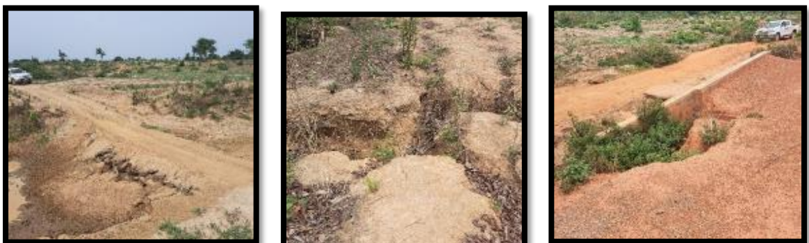
Plate 4. 3: Pictures Showing Current Status of 7Km Kuyi – Kampala Road Corridor
