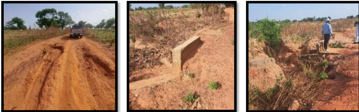
Plate 4. 2: Pictures Showing Current Status of 3Km Kontagora-Gangaren Sagi Road
