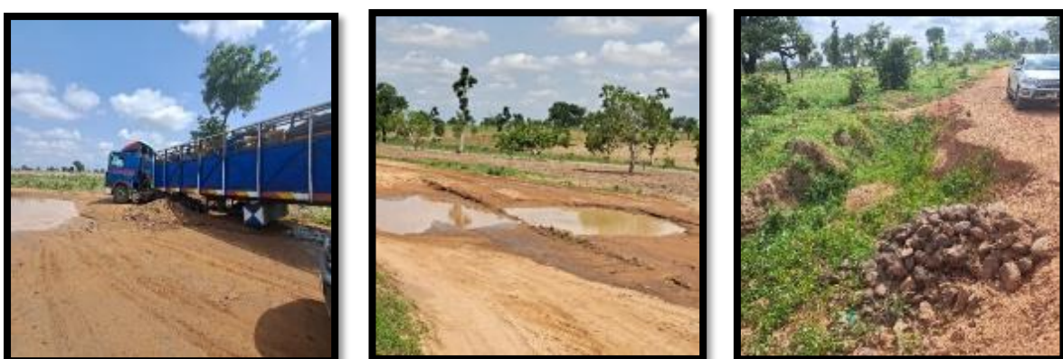
Plate 4. 4: Pictures Showing Current Status of 35Km Beji-Makera-Jangara Road
