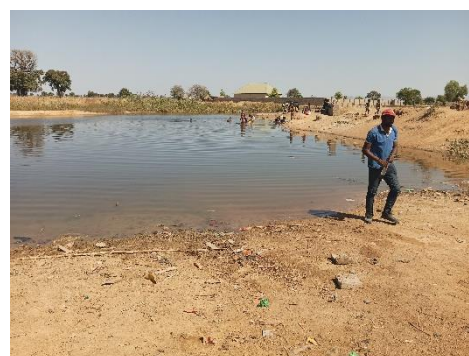
Existing earth Dam (source from Yadzaram River) source of water to the school
