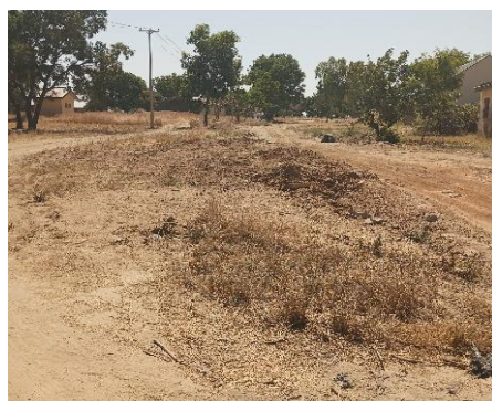
Existing access road to be rehabilitated
