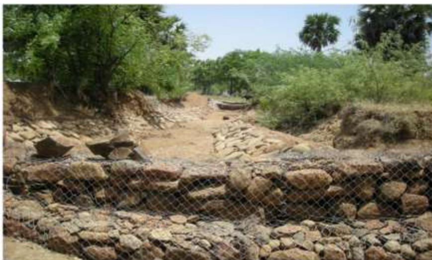
Plate 4.8: Gabion Check Dam to counter erosion
