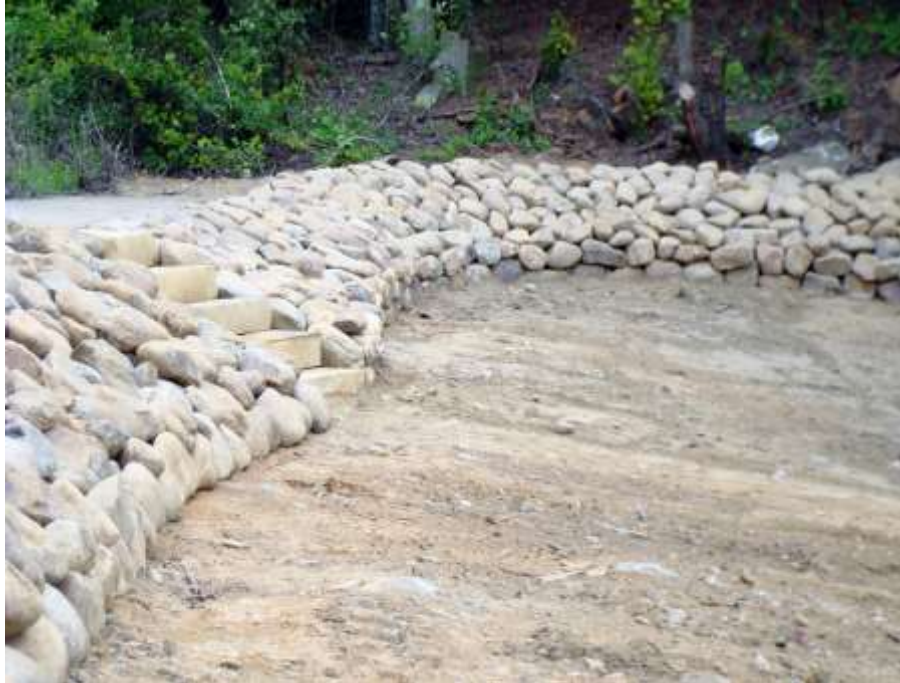
Plate 4.9 River Rock Riprap for Stream Bank Erosion Control
