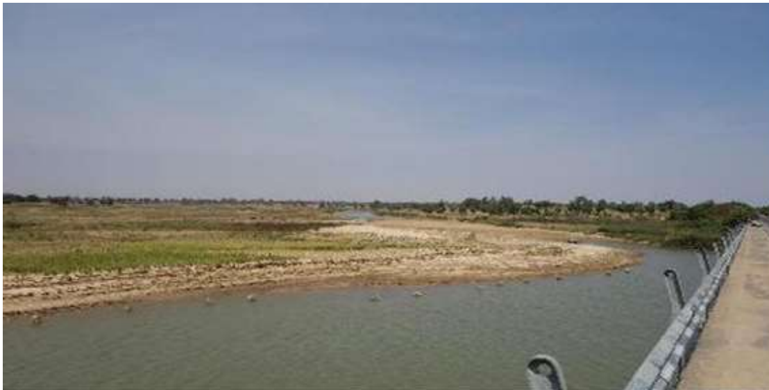
Plate 3.7 Siltation at the Kano Water Treatment Plant Panshekara
