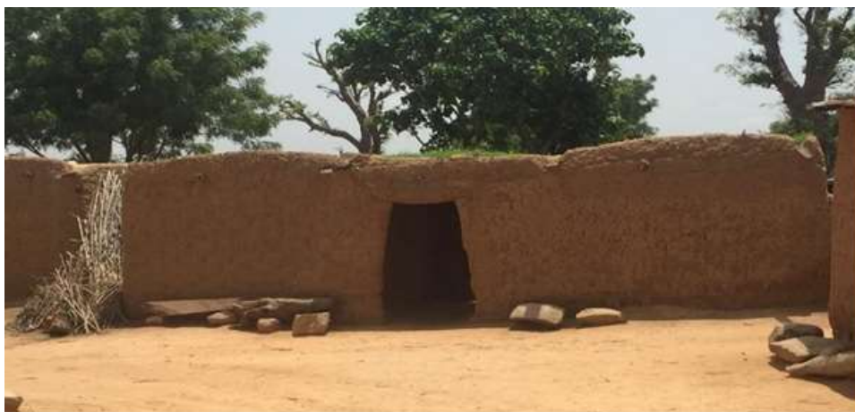
Plate 5.10.: A typical building made of wood, sand and grasses in the project site
