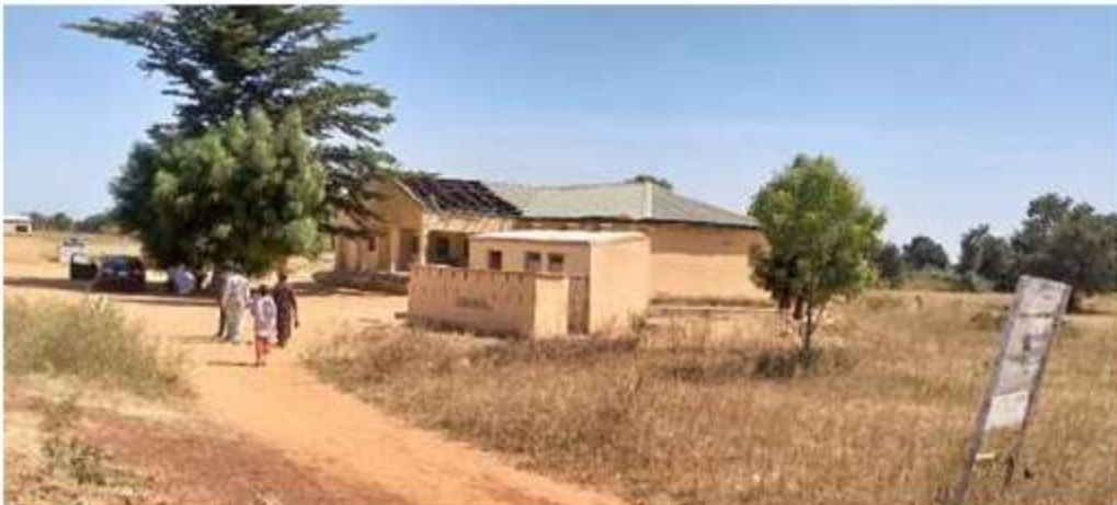
ate 5.14: Laterite surface road Traversing a village area
