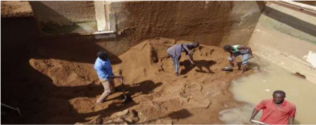
Plate 3.6: Evidence of manual evacuation of Sand deposits at Challawa Water Works Treatment plant at Panshekara for kano Municipality.
