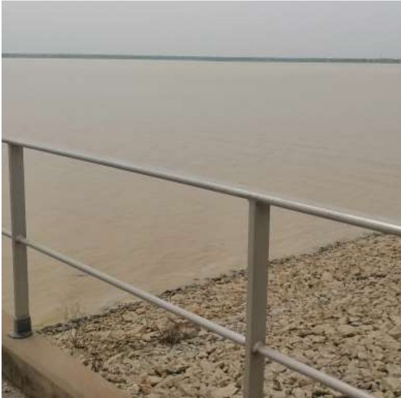
Plate 4.4. A view of the Challawa Gorge Dam Reservoir
