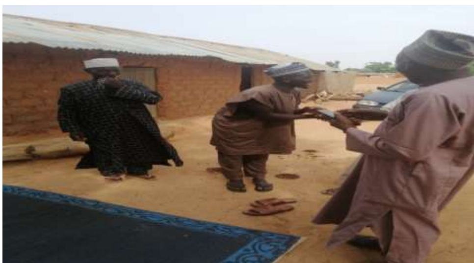
Plate 5.11.: A typical building made of sand and corrugated iron sheets at the Dam site Area.
