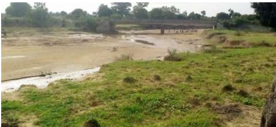
Plate 4.3: Challawa River Bank degradation and destruction of critical infrastructure
